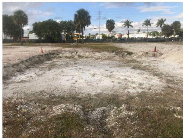
Photograph 2. View towards the north showing the SS-1 Excavation (still opened) in the northern portion of the subject site.
