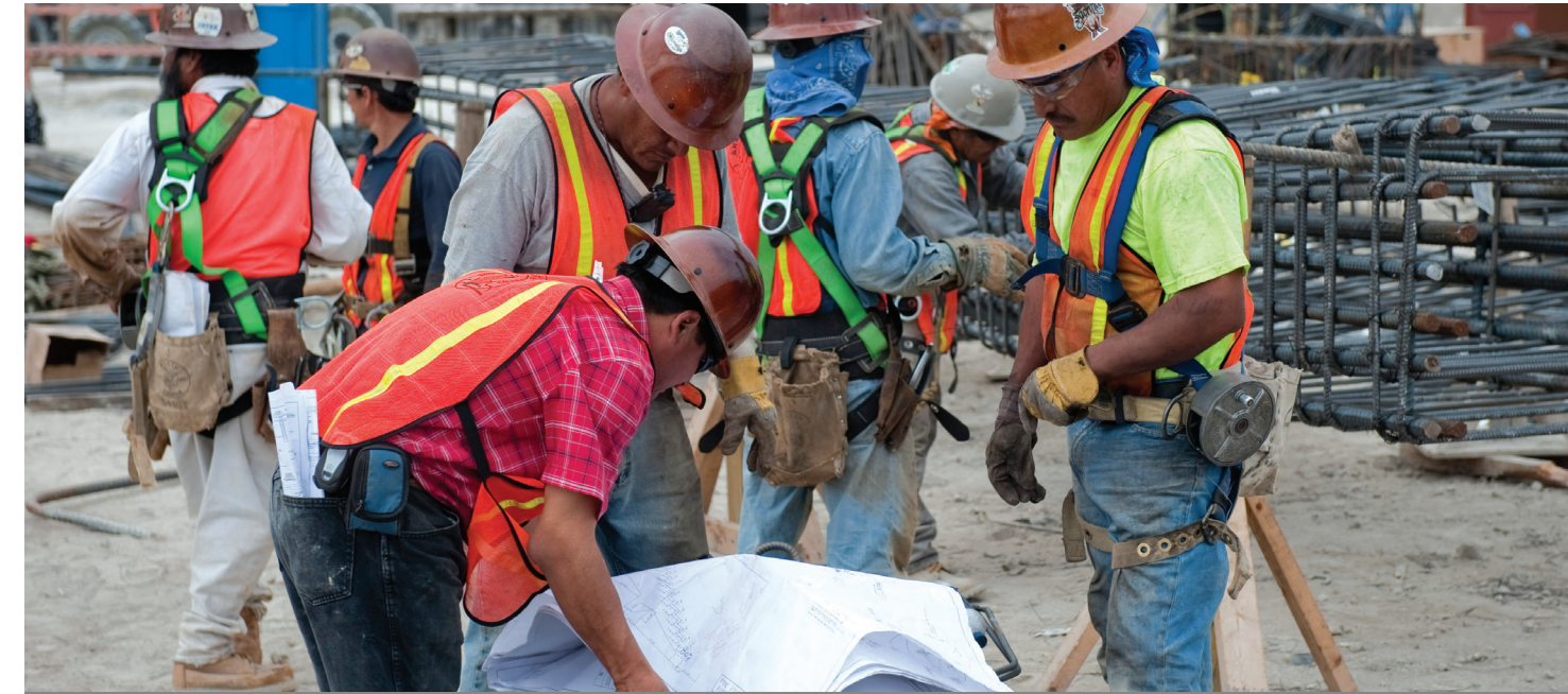
A new Florida Marlins Baseball Ballpark is under construction with a sustainability approach. The ballpark will be accessible via public transportation, will have solar panels on its parking garages, will have accessible seating, and will be applying for Leadership in Energy and Environmental Design (LEED) Silver certification. Five thousand constructions jobs are projected by the end of the project and once the Ballpark is open, 2,550 full and part-time jobs are anticipated.
