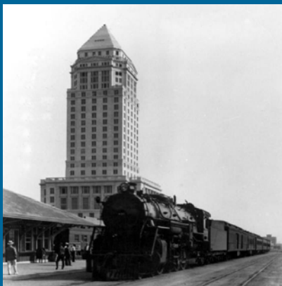
The Past: The FEC Miami Railroad Station
