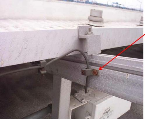
Improper Cad Tek screw used to hold lug Wrong connectors
