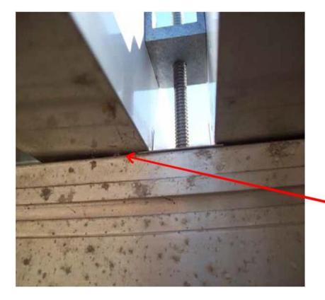
Notice slight gap caused by properly installed clip.
