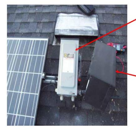
NEMA 3R disconnect on sloped roof designed for vertical mounting only
