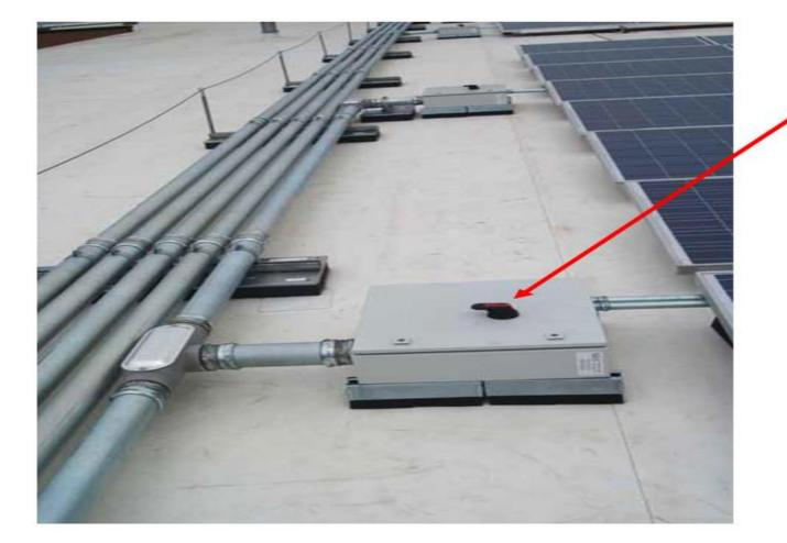
NEMA 4 Combiner Box with disconnect built-in. Designed for horizontal or vertical mounting
