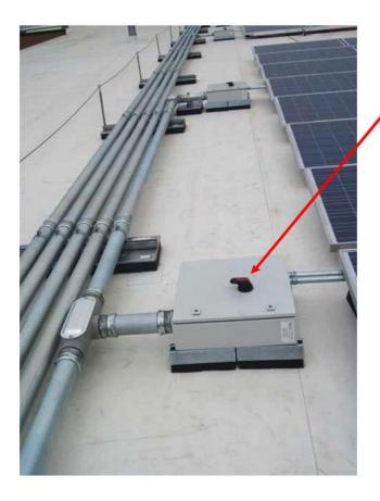
NEMA 4 **Combiner Box** with disconnect built-in. Designed for horizontal or vertical mounting
