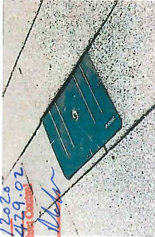
2. INSERT THE FLASHING SO THE TOP PART IS UNDER THE NEXT ROW OF SHINGLES AND THE HOLE LINES UP WITH THE PILOT HOLE.
