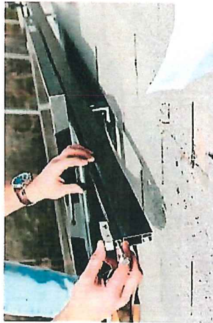
1. SLIDE END CLAMP ON TO RAIL BY ENGAGING THE TWO T-GUIDE BRACKETS WITH THE TOP SLOT OF THE RAILS. SLIDE END CLAMP ASSEMBLY ON TO RAIL UNTIL BOLT HEAD ENGAGES WITH END OF RAIL.
