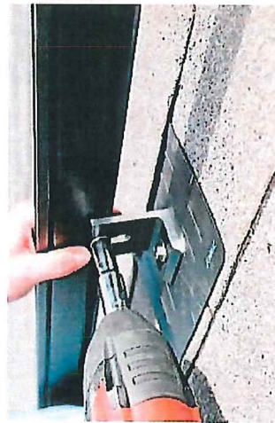
7. USE DRILL TO TIGHTEN NUT ONTO T-BOLT.
