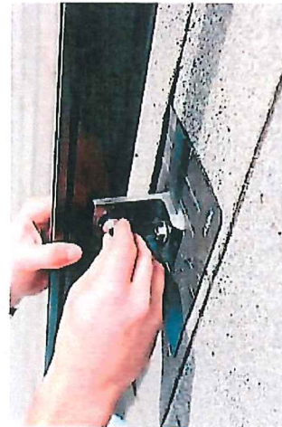
6. HAND TIGHTEN NUT UNTIL RAIL ALIGNMENT IS COMPLETE. VERIFY THAT POSITION INDICATOR ON BOLT IS VERTICAL (PERPENDICULAR TO RAIL).
