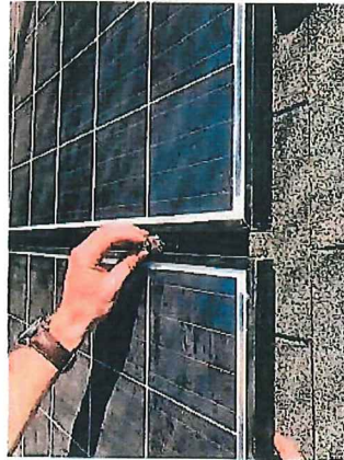
4. INSERT 1/4" T-BOLT INTO RAIL
