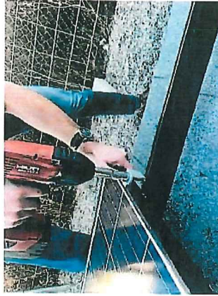
2. ENGAGE MODULE FRAME WITH ENDCLAMP. TIGHTEN T-BOLT WITH DRILL.
