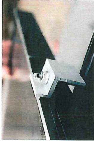
3. SEE MODULE ENGAGED BY ENDCLAMP.
