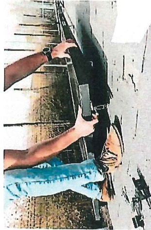
2. INSTALL THE FIRST END MODULE ONTO RAILS WITH THE FLANGE OF THE MODULE FRAME POSITIONED BETWEEN END CLAMPS AN ENDS OF RAILS.
