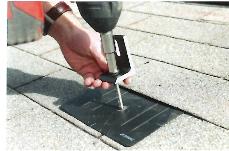
3. INSERT THE LAG BOLT THROUGH THE L-FOOT IN THE ORDER SHOWN IN THE IMAGE. VERIFY PROPER ORIENTATION BEFORE TIGHTENING LAG BOLTS.
