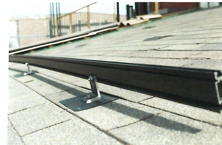
8. SEE RAIL ATTACHED TO L-FOOT.
