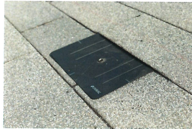
2. INSERT THE FLASHING SO THE TOP PART IS UNDER THE NEXT ROW OF SHINGLES AND THE HOLE LINES UP WITH THE PILOT HOLE.
