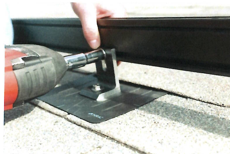
7. USE DRILL TO TIGHTEN NUT ONTO T-BOLT.
