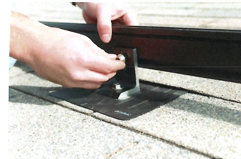
6. HAND TIGHTEN NUT UNTIL RAIL ALIGNMENT IS COMPLETE. VERIFY THAT POSITION INDICATOR ON BOLT IS VERTICAL (PERPENDICULAR TO RAIL).
