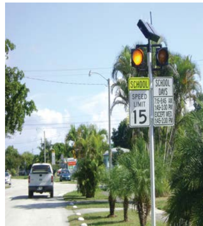
Solar Flashing School Zone Signal
