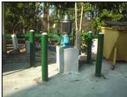
Ground Water Intake
