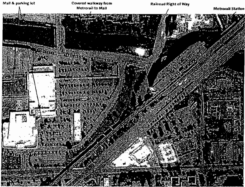
Existing Conditions near Railroad Right-of-Way
