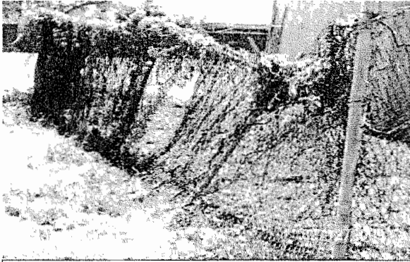
Damaged fencing (Area B1)
