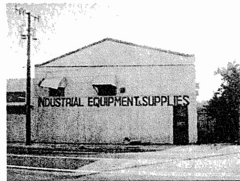
Property at 2055 NW 7 th Avenue with partially boarded up windows to the site and stained (Area A1)
