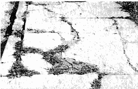
Cracked sidewalks (Area B2)
