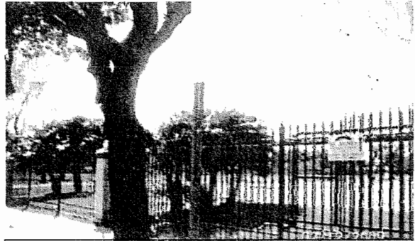
Missing street signage (Area A1)
