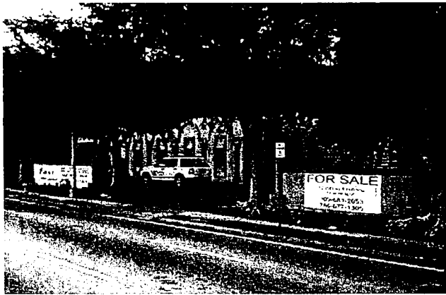
Commercial for sale and structure deterioration located on 15700 NW 7 th Avenue.
