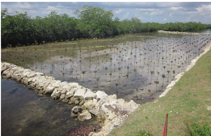
A newly constructed earthen plug along Card Sound Road will help limit salt water intrusion
