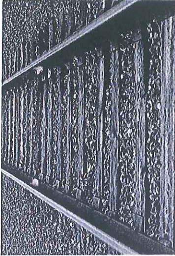
Steel railroad rail embedded flush with concrete
