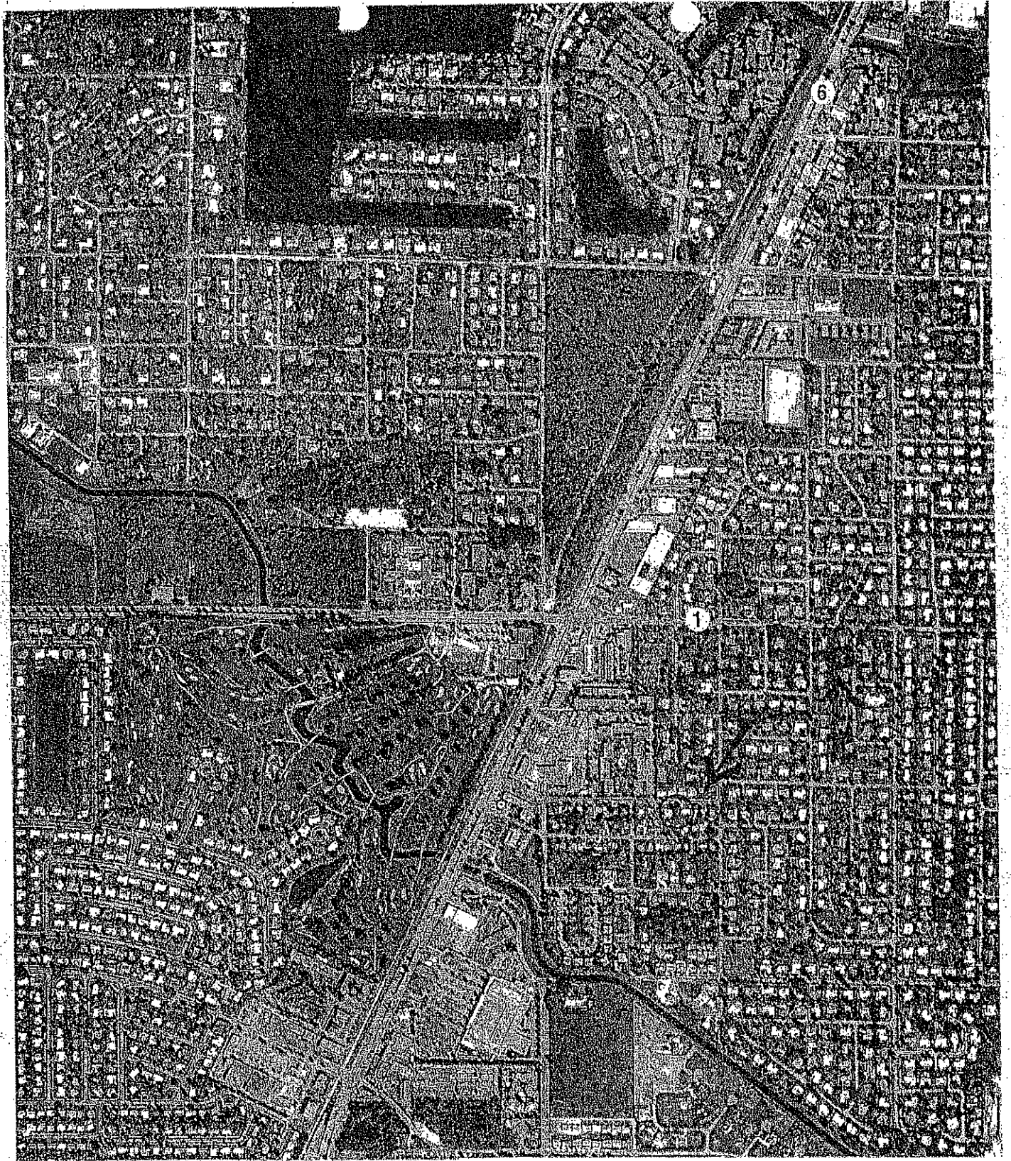
1990s aerial photograph showing suburban development in the Rockdale area. The former sloughs are now canals. The last remaining pinelad track is the triangular area between Coral Reef Drive and Mitchell Drive (location of the old FEC quarry). Mr. Troeger's house is within the circled area.
