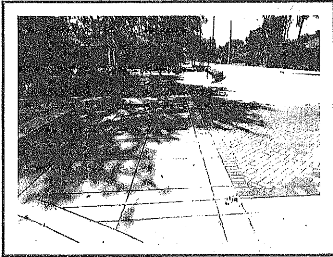
Completed SW 59 th Place Infrastructure Repairs
