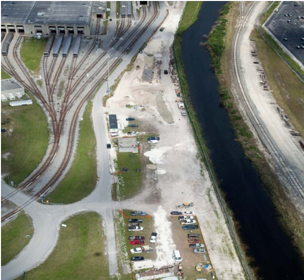
Test Track – southern portion looking north
