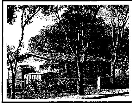
Completed Roofing Work
