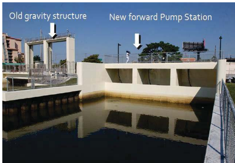
Figure 18: Adaptation of the District's gravity-based water management infrastructure
