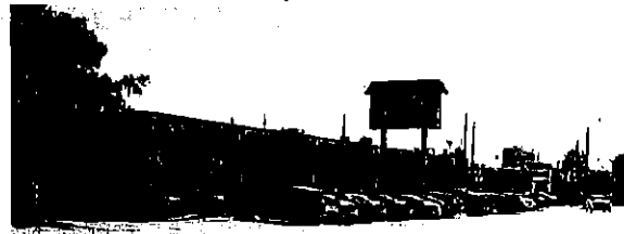
West Dixie Highway looking South from Snake Creek Canal Bridge
