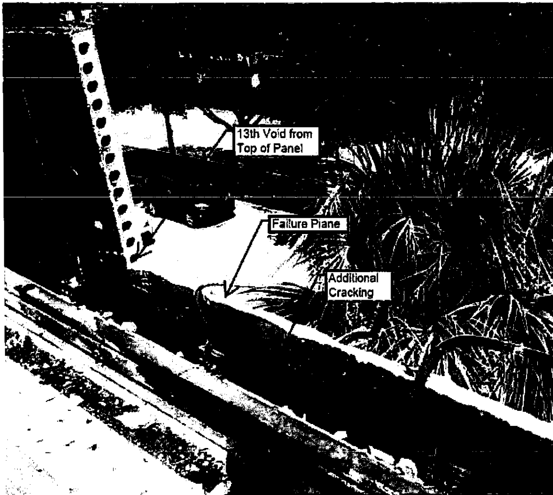
Figure 3: Type "B" Acoustical Barrier Panel Failure Plane
