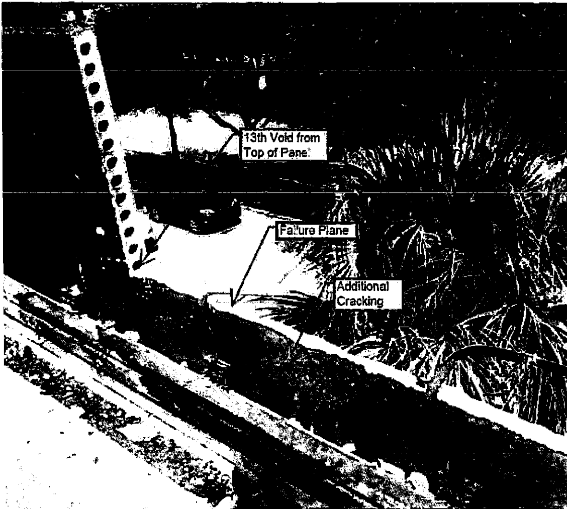
Figure 3: Type "B" Acoustical Barrier Panel Failure Plane
