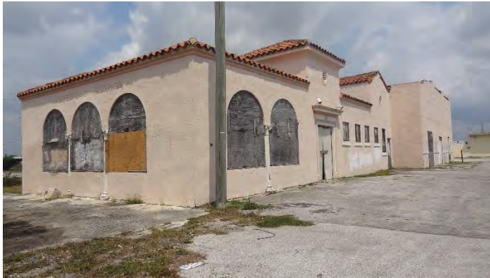
Figure 8: The Homestead Train Station is boarded up and vulnerable
