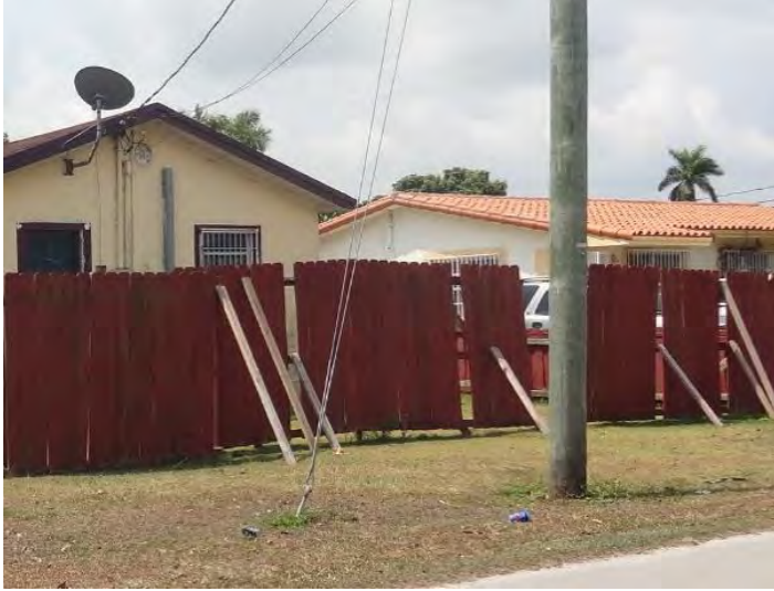
Figure 9: Damaged properties are evident
