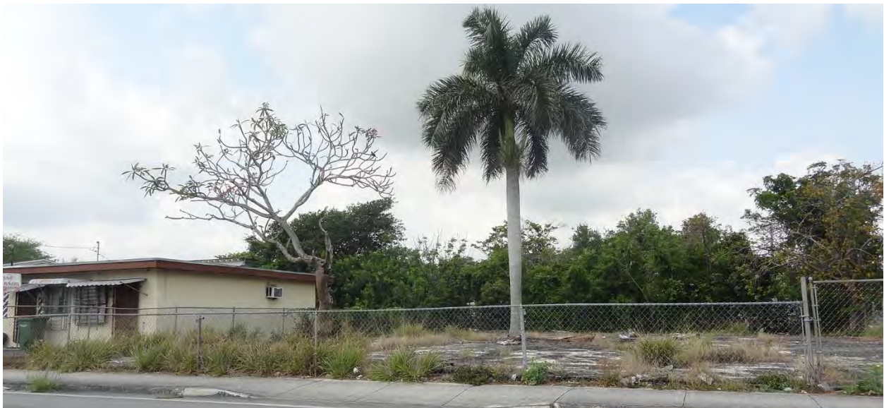
Figure 10: Building and Site Deterioration
