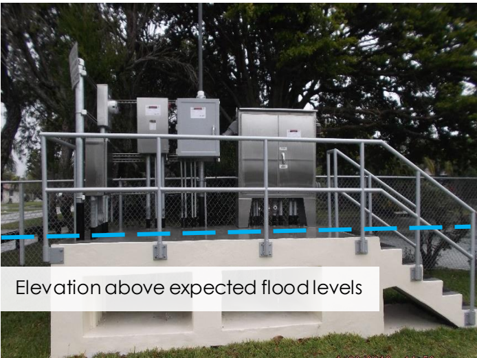
Figure 23: Electrical panels are elevated on a four-foot pad to protect them from flooding
