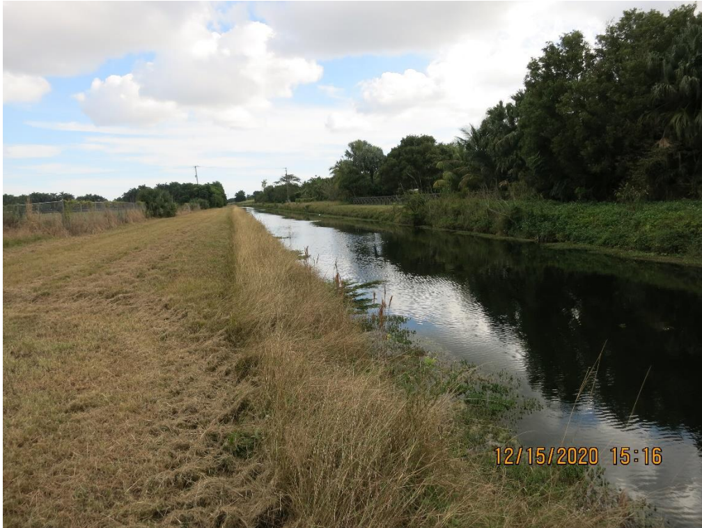
View east along north bank of C-103 Canal
