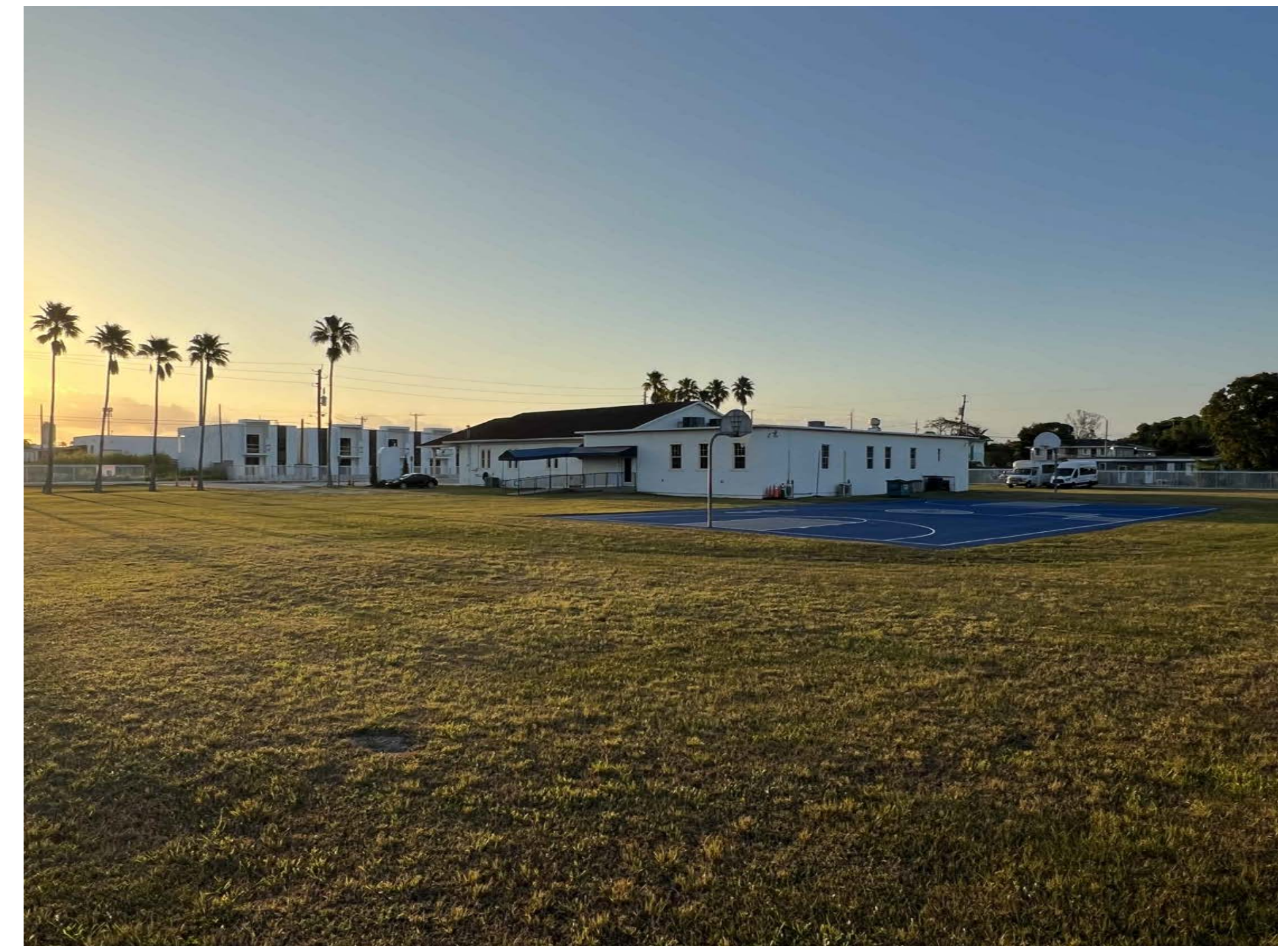
NORTH SIDE FACADE & REAR WEST FACADE
