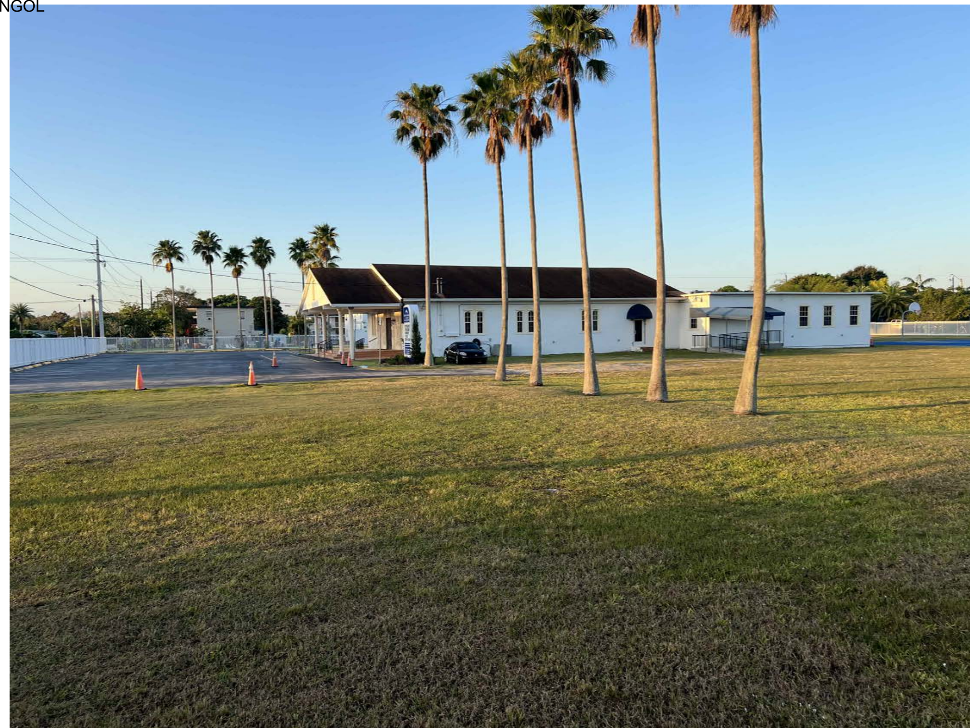
PROPERTY NORTH SIDE FACING 169TH STREET
