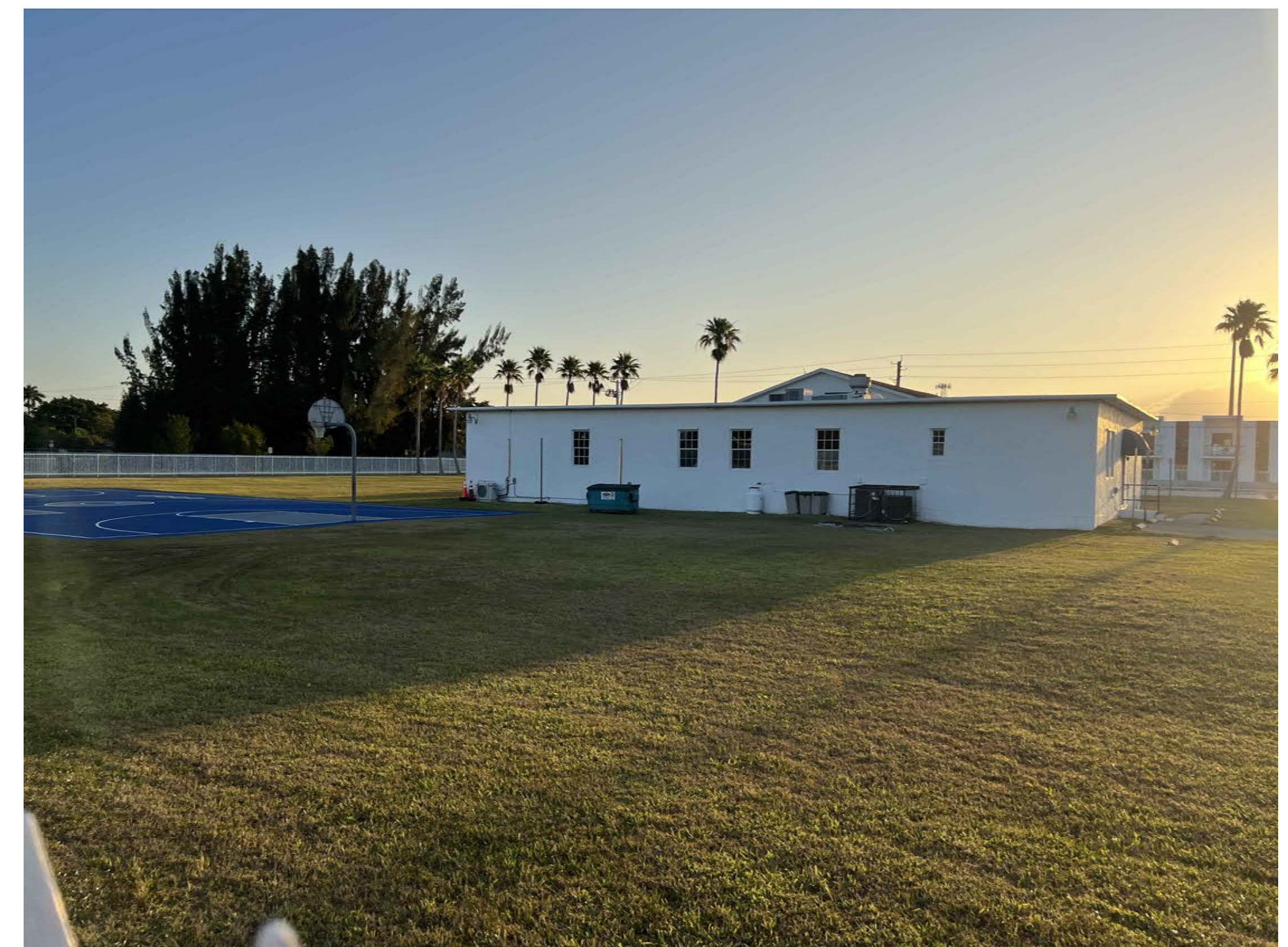
REAR WEST FACADE
