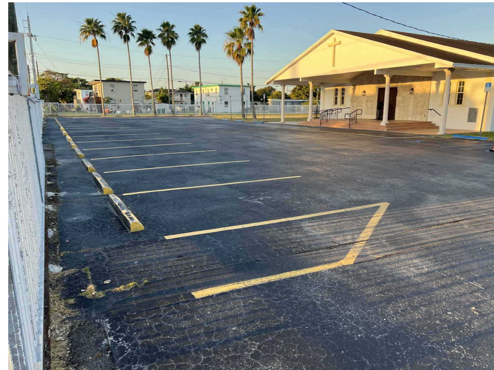
FRONT EAST FACADE FACING 100TH AVE
