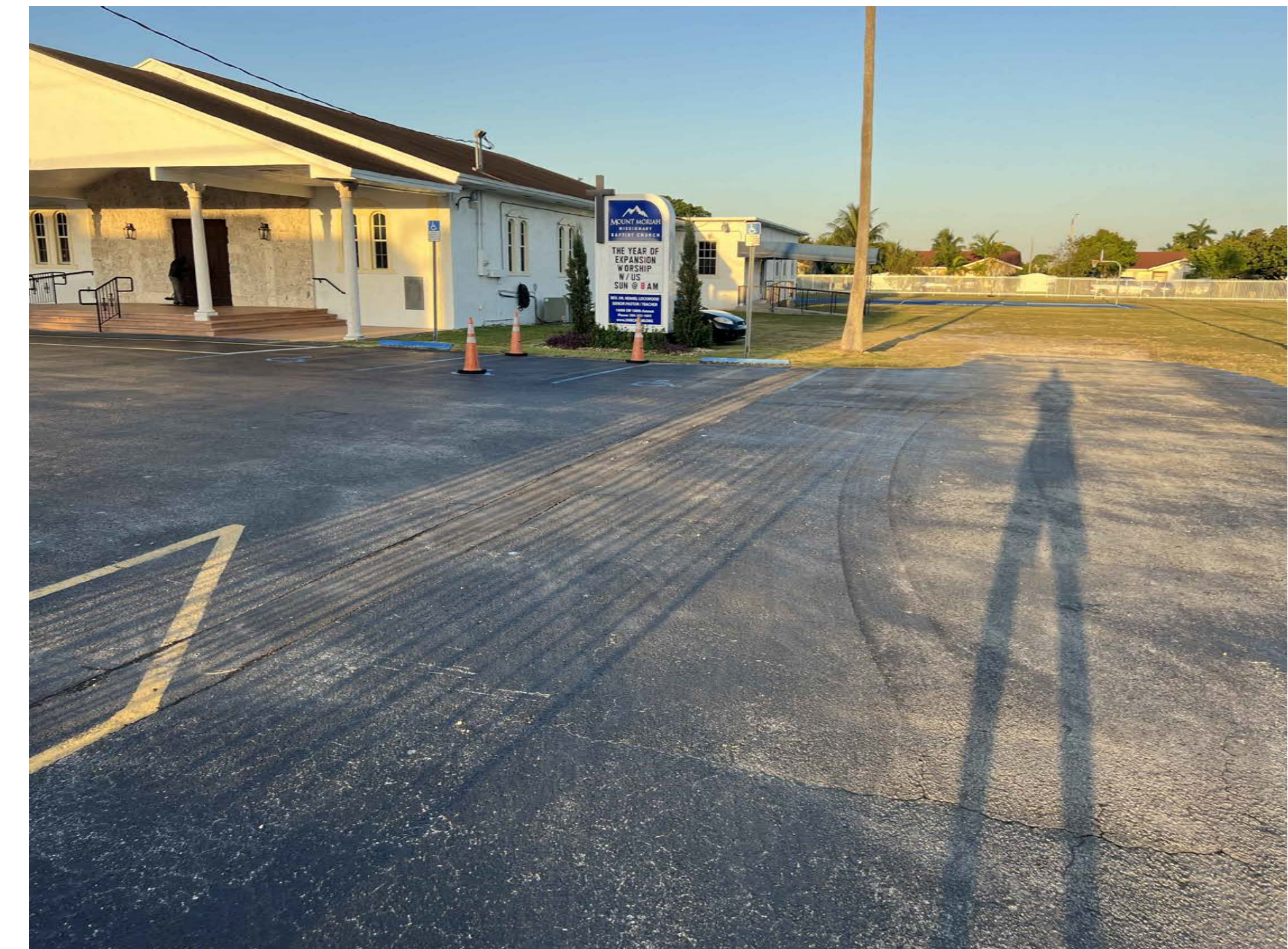
PARTIAL FRONT EAST FACADE FACING 100TH AVE AND NORTH SIDE
