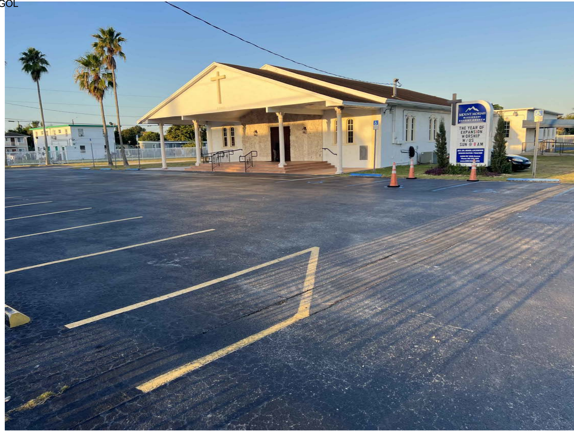
FRONT EAST FACADE FACING 100TH AVE
