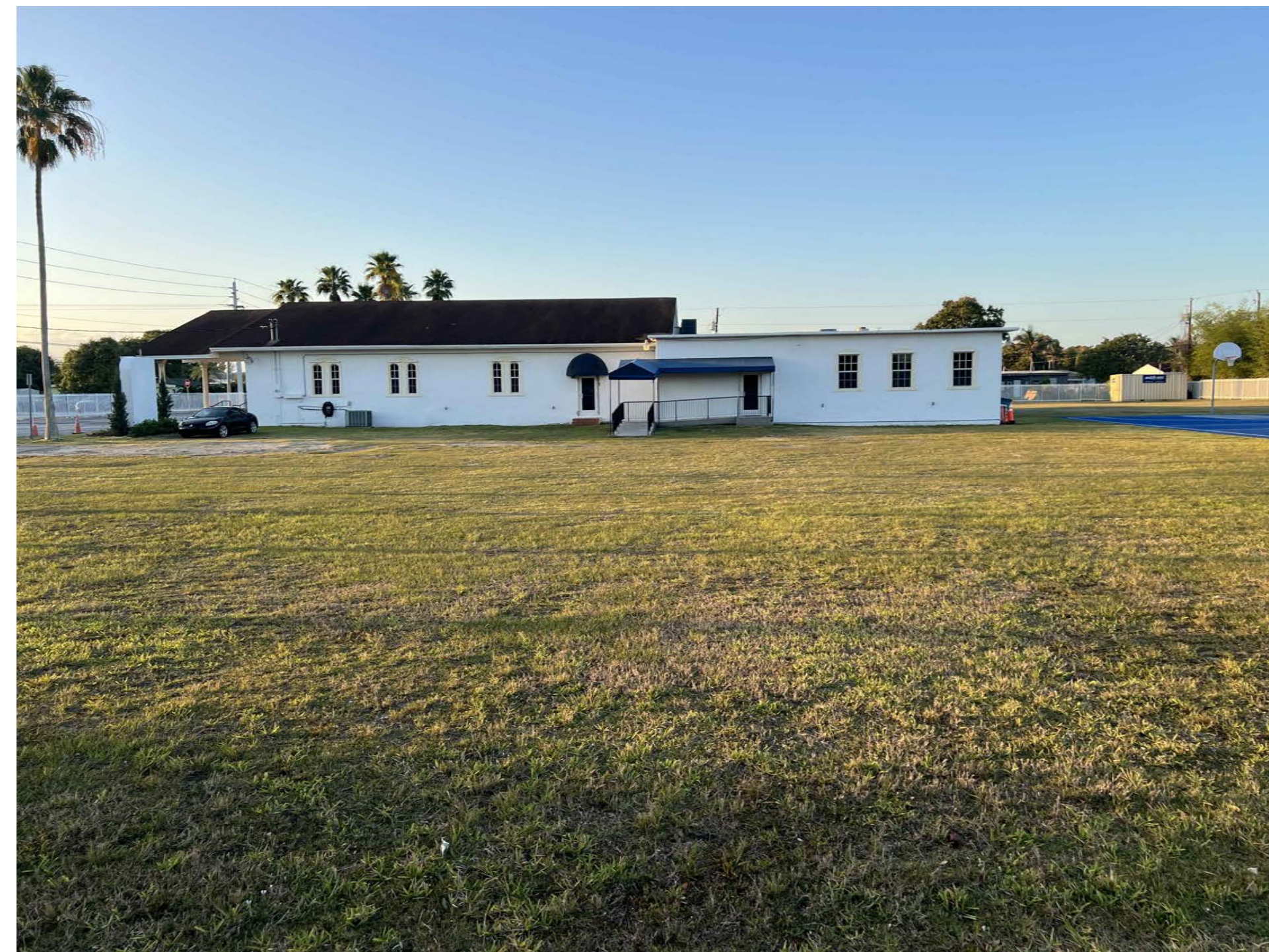
PROPERTY NORTH SIDE FACING 169TH STREET
