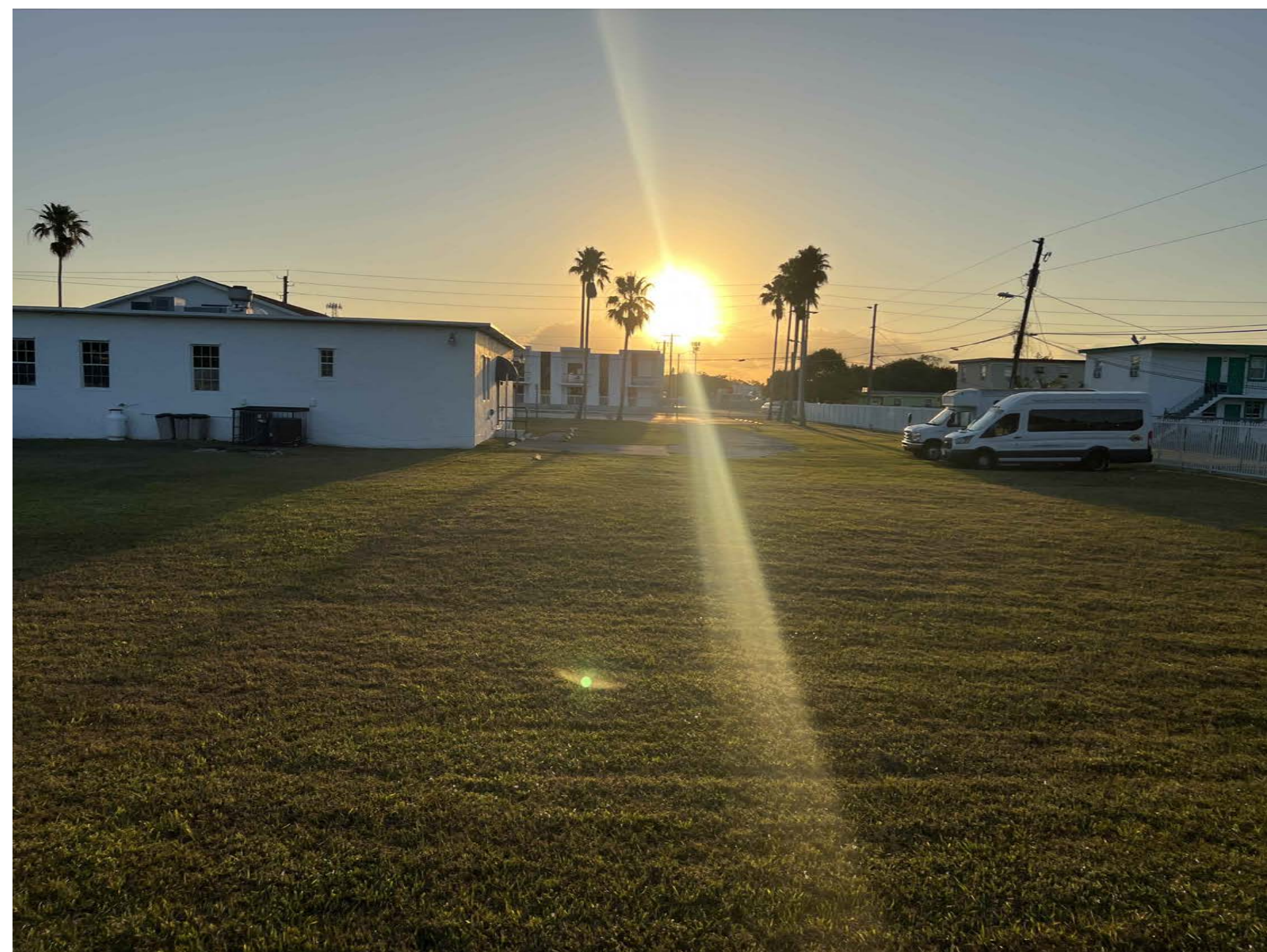
SOUTH SIDE PROPERTY AREA & PARTIAL REAR WEST FACADE
