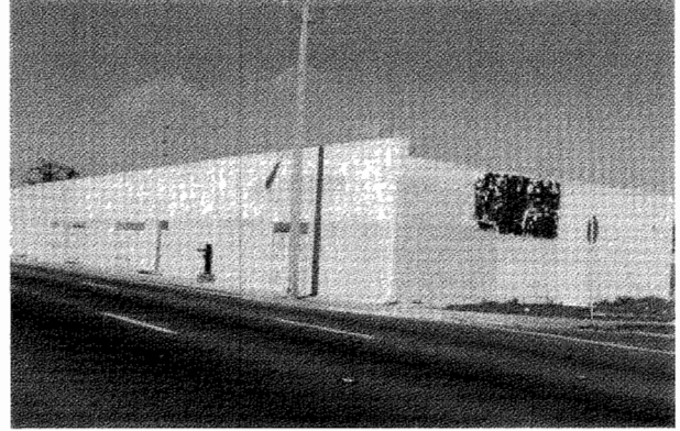
Abandoned building with blocked entrances on 22 nd Avenue north of 86 th Street
