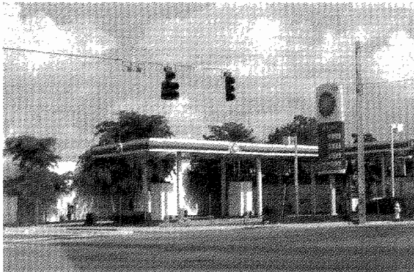
Commercial vacant property (BP gas station) located on north west corner of 22 nd Avenue and 62 nd Street
