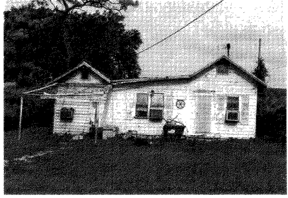
Dilapidated property on 10 th Court north of 79 th Street with worn paint and caved roof
