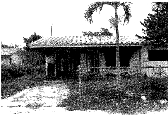
Dilapidated property near Liberty City
