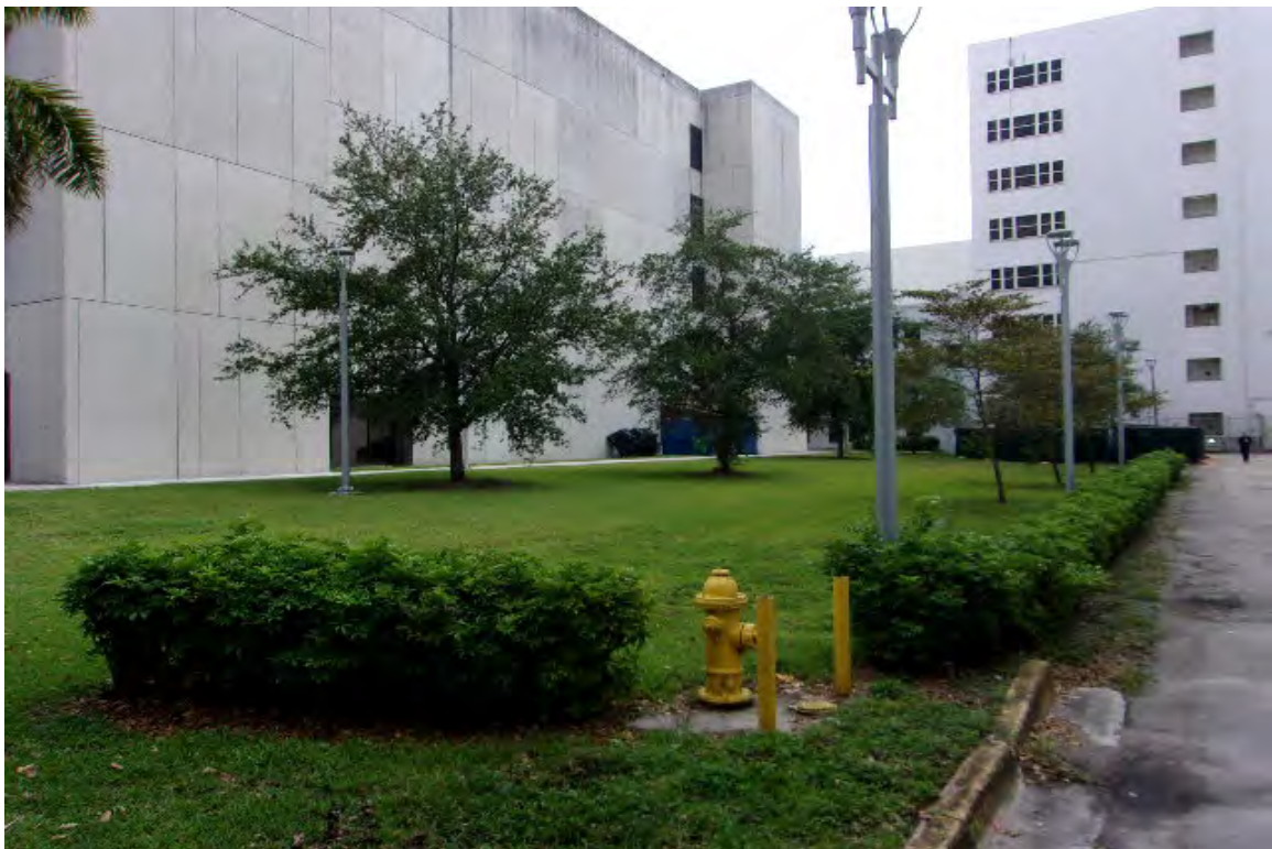
LOOKING NORTHEASTERLY AT SUBJECT
