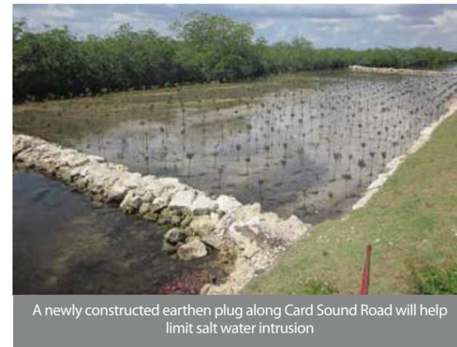
A newly constructed earthen plug along Card Sound Road will help limit salt water intrusion
