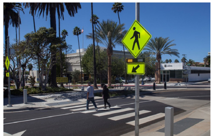
A marked crosswalk with Rectangular Rapid Flashing Beacon indications creates a significantly safer environment.
