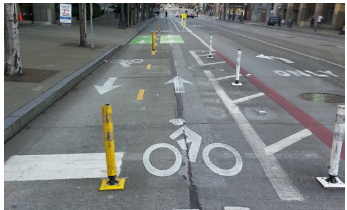
Implementation often can be achieved through restriping and flexible traffic delineators without full reconstruction.
