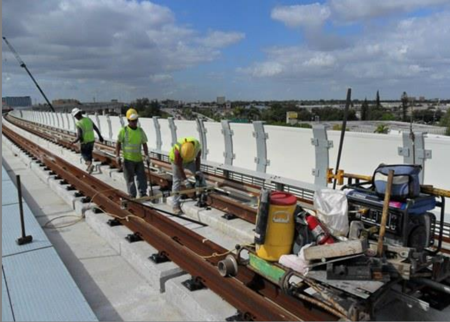
Running rail alignment
