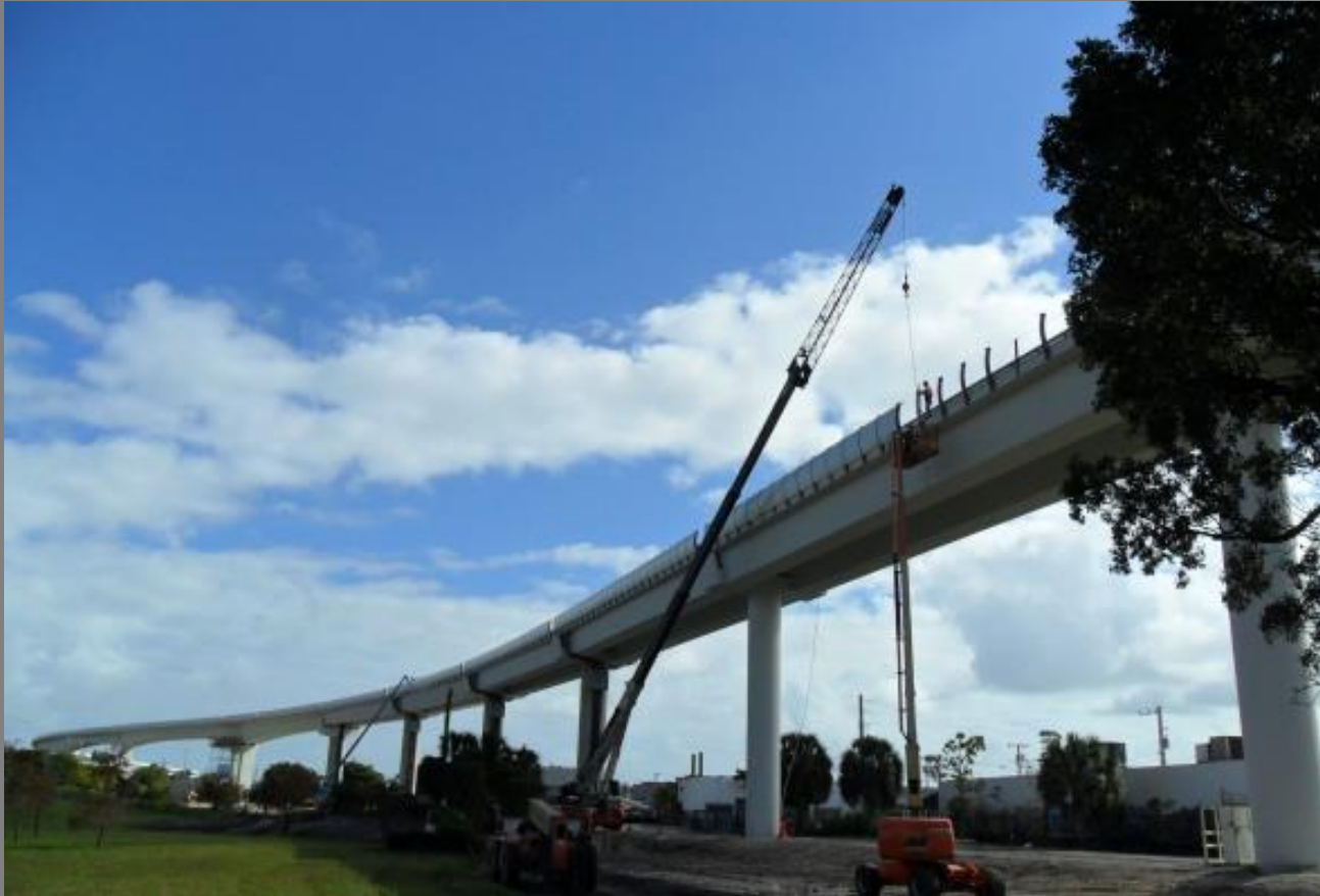
Installation of sound wall panels
