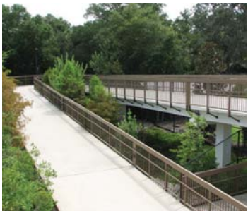
ADA accessible ramp to pedestrian bridge
