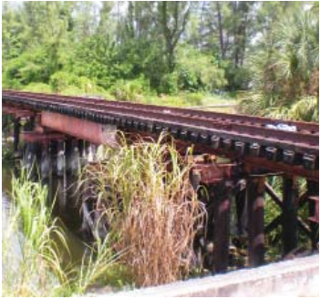
Tamiami C-4 Canal Bridge
