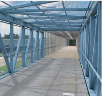
'Caged' bridge structure
