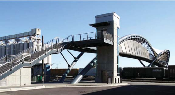
Iconic pedestrian bridge in Seattle, Washington
