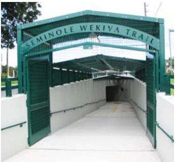
Hwy 434 tunnel entrance ramp and gate
