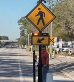
Push button activated stutter signal (flashing beacon)
