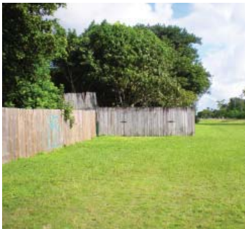
Residential fence encroachment
