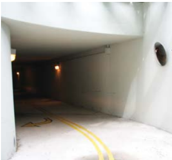
Hwy 434 tunnel entrance
