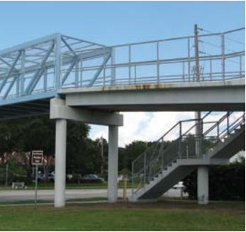
Ramp approach to bridge with stairs
