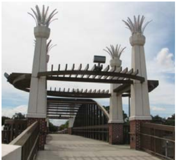
Iconic bridge along West Orange Trail
