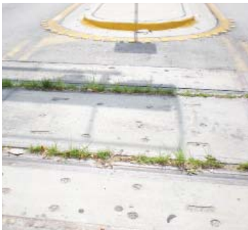
West Flagler St. existing tracks
