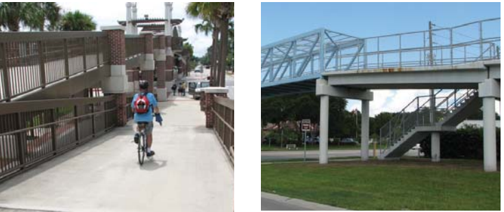
Above-Grade crossing in Apopka, Florida
