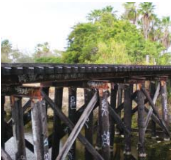
Coral Gables C-3 Canal Bridge
