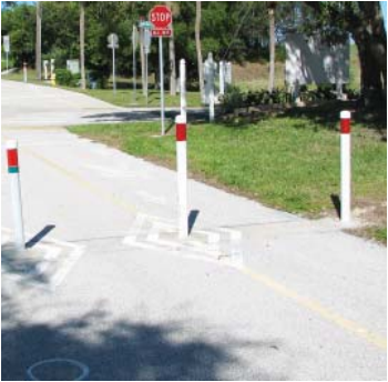
Bollards at controlled entrances
