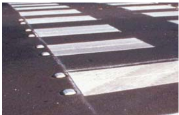
Example of well defined crosswalk markings
