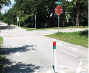
Bollards at each At-Grade crossing
