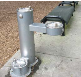
Example of ADA accessible drinking fountain
