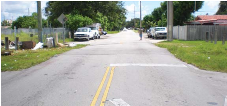
SW 12th St. existing local street crossing
