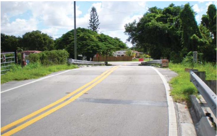
North Waterway Drive with no sidewalk access
