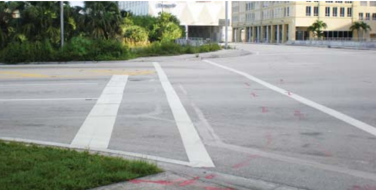
SW 85th St. with existing striped crosswalk
