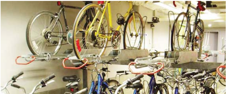
Indoor bike storage facilities
