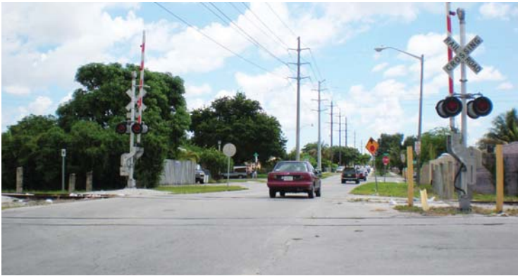
SW 4th St. existing railroad crossing
