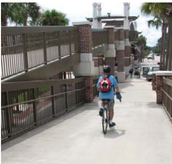
ADA accessible ramps for Above-Grade crossing
