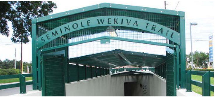
Seminole Wekiva Trail Below-Grade crossing tunnel entrance
