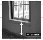
be required in adjoining areas of the basement. Where emergency escape and rescue openings are provided, they shall have a sill height of not more than 44 inches above the floor.
