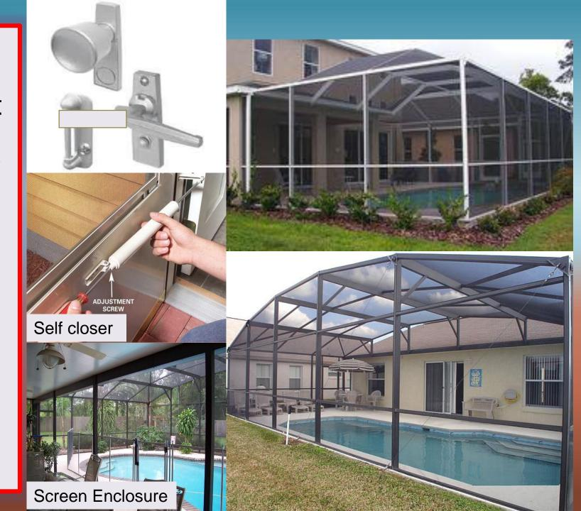
R4501.17.1.12 The barrier must be placed around the perimeter of the pool and must be separate from any fence, wall, or other enclosure surrounding the yard unless the fence, wall, or other enclosure or portion thereof is situated on the perimeter of the pool, is being used as part of the barrier, and meets the barrier requirements of this section
