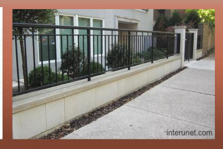
• **R4501.17.1.4** Where the barrier is composed of horizontal and vertical members and the distance between the tops of the horizontal members is less than 45 inches (1143 mm), the horizontal members shall be located on the swimming pool side of the fence. Spacing between vertical members shall not exceed 1 3/4 inches (44 mm) in width. Where there are decorative cutouts within vertical members, spacing within the cutouts shall not exceed 1 3/4 inches (44 mm) in width.
