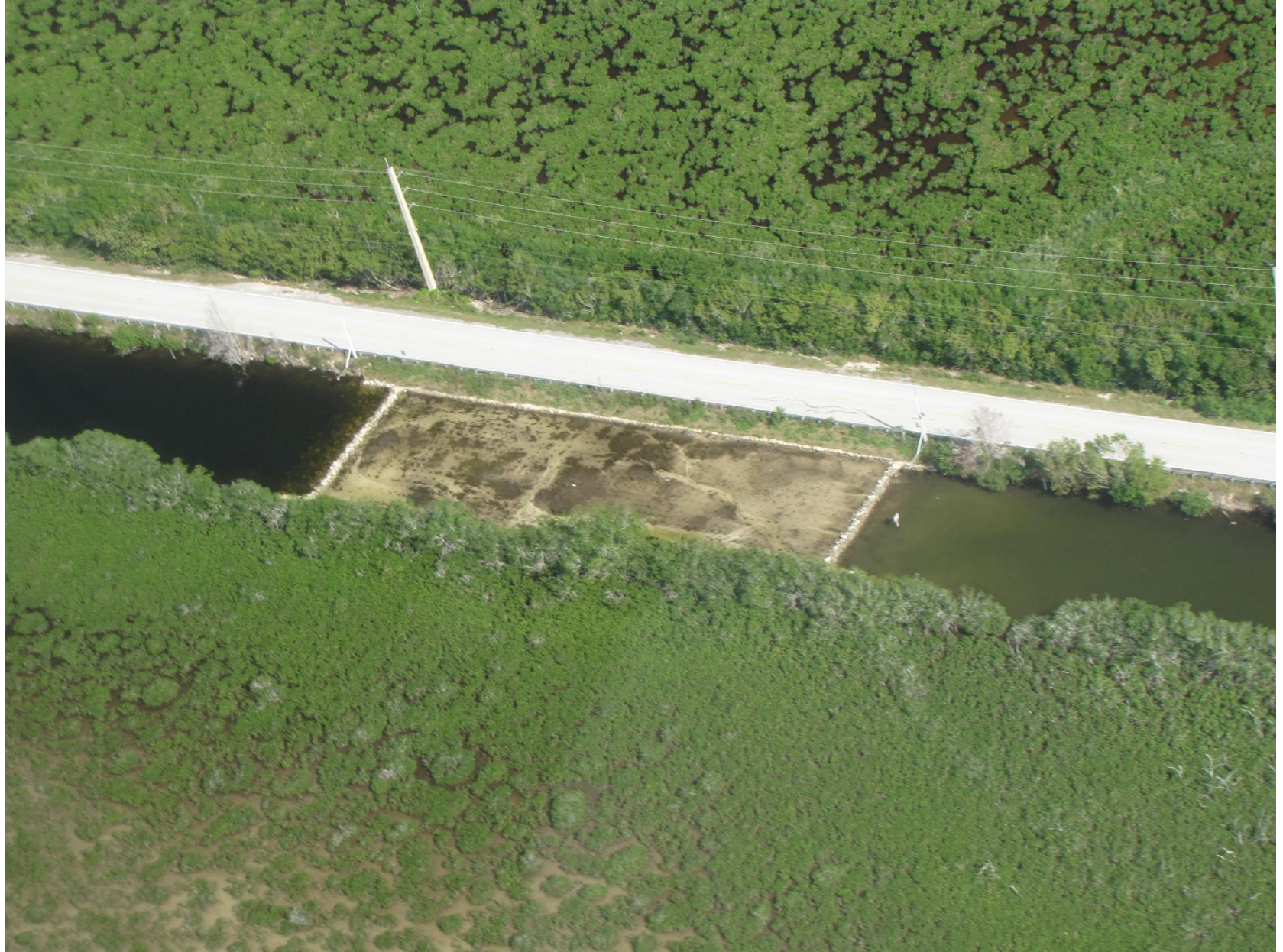
CONSTRUCTED PILOT PROJECT CARD SOUND ROAD BORROW CANAL PLUG
