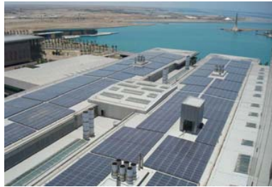
ROOF TOP SOLAR PANEL ARRAY
