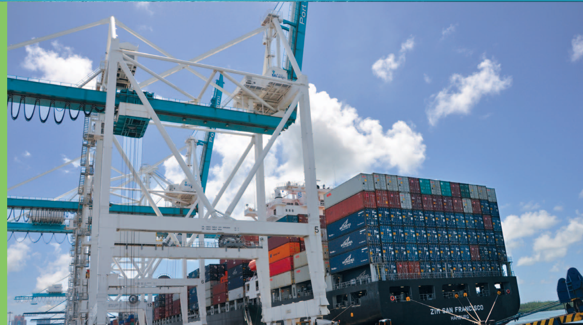
State-of-the-art super post-panamax gantry cranes
