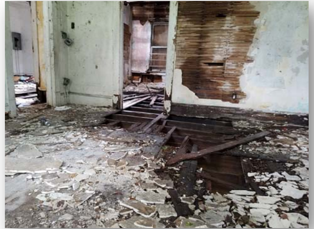
Beam and Floor Damage
