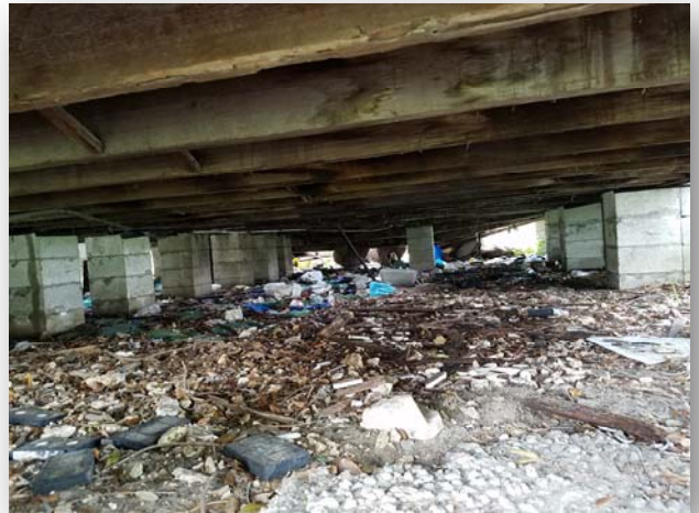
Rotten Main Beams/Center Missing Support
