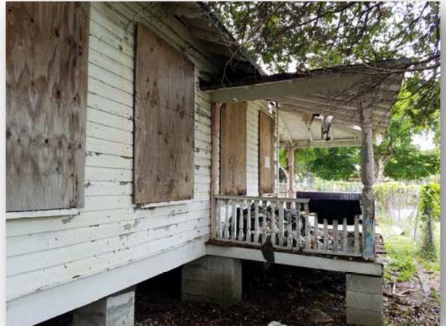
West Side of Building
