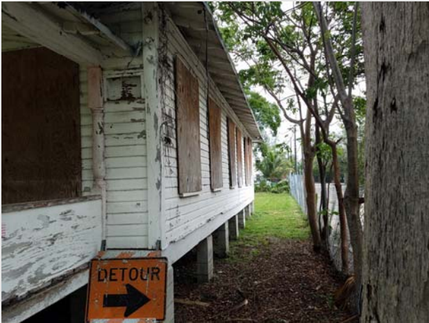
East Side of Building
