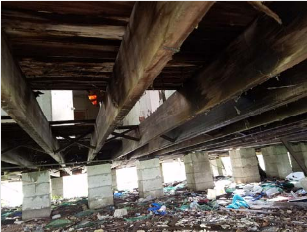
Damage to floor beam support
