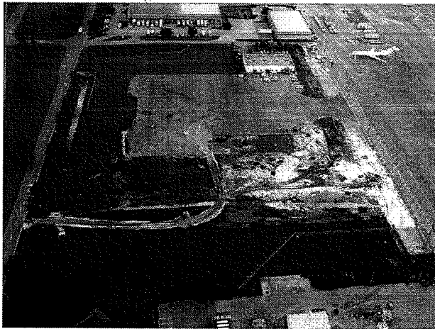
T-553 Site at MCO under construction.
