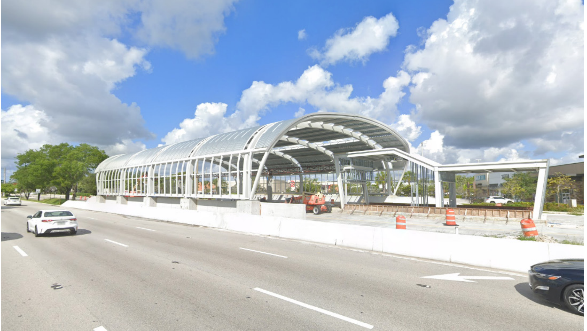
Figure 5-5: South Corridor Station Under Construction
