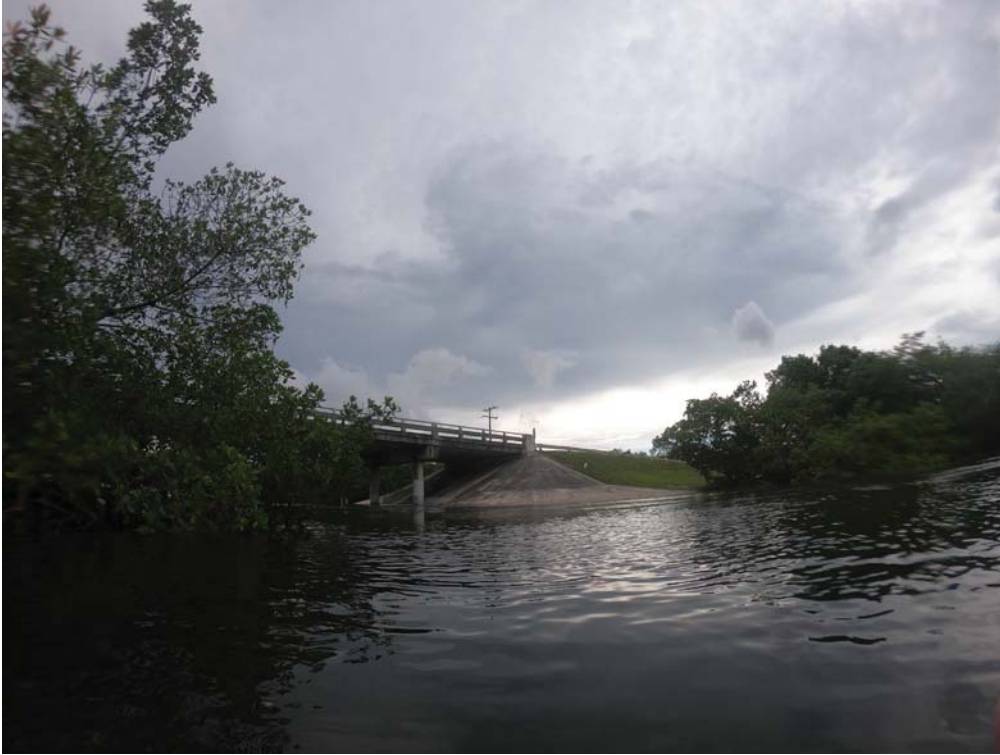
Photo 1 View of the existing bridge, facing northeast.
