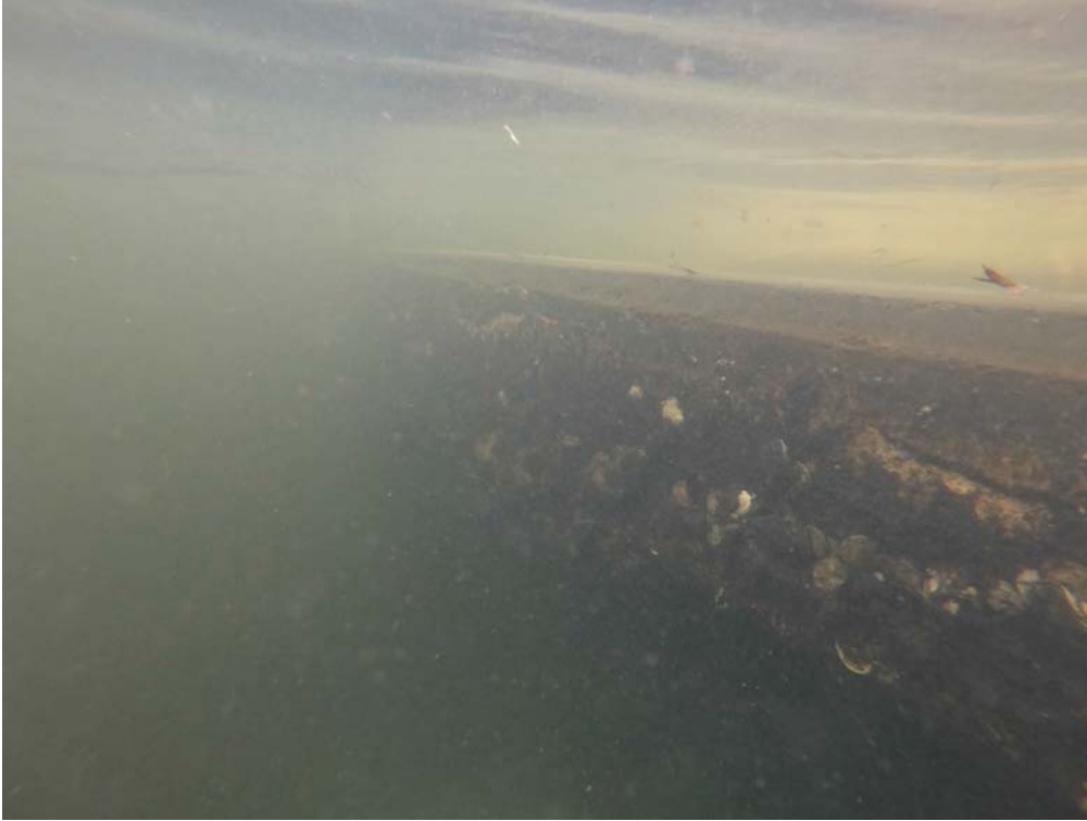
Photo 3 Typical view of oyster growth on existing bridge.
