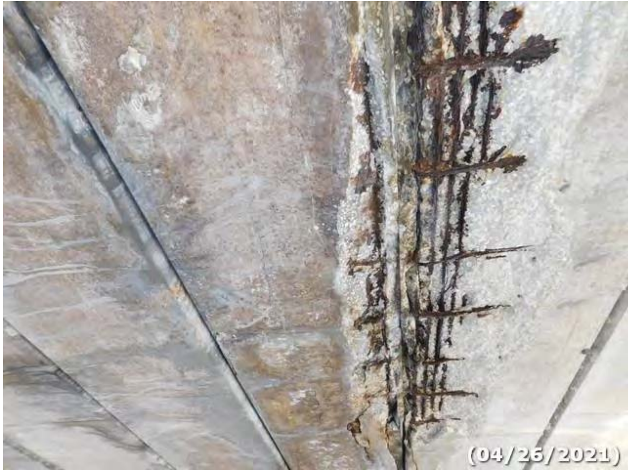
Photo 06 Element/Env 8099/3: PS Conc Slab (Sonovoid)
