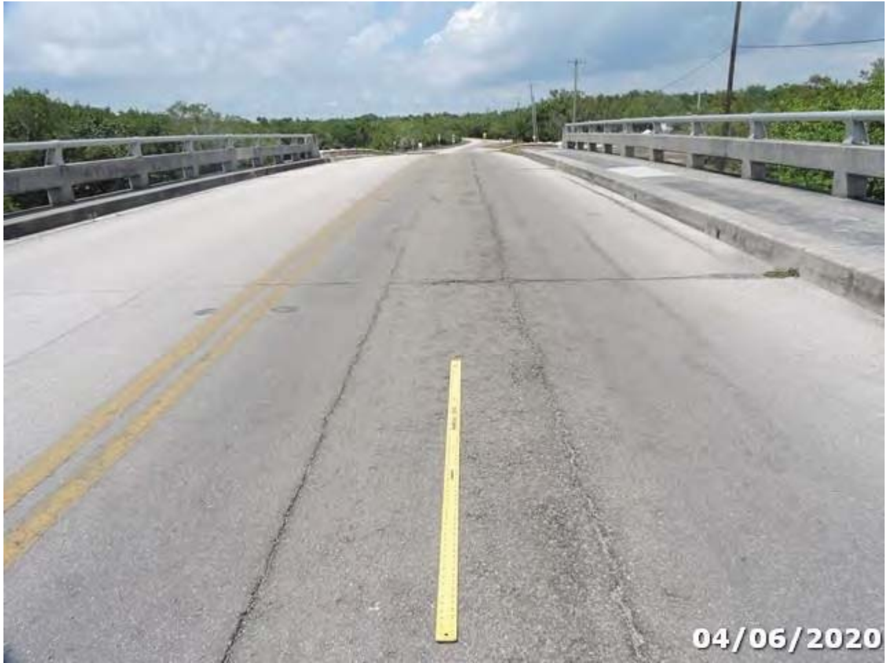
Photo 12 Element/Env 8099/ 510/3: PS Conc Slab (Sonovoid)/ Wearing Surfaces
