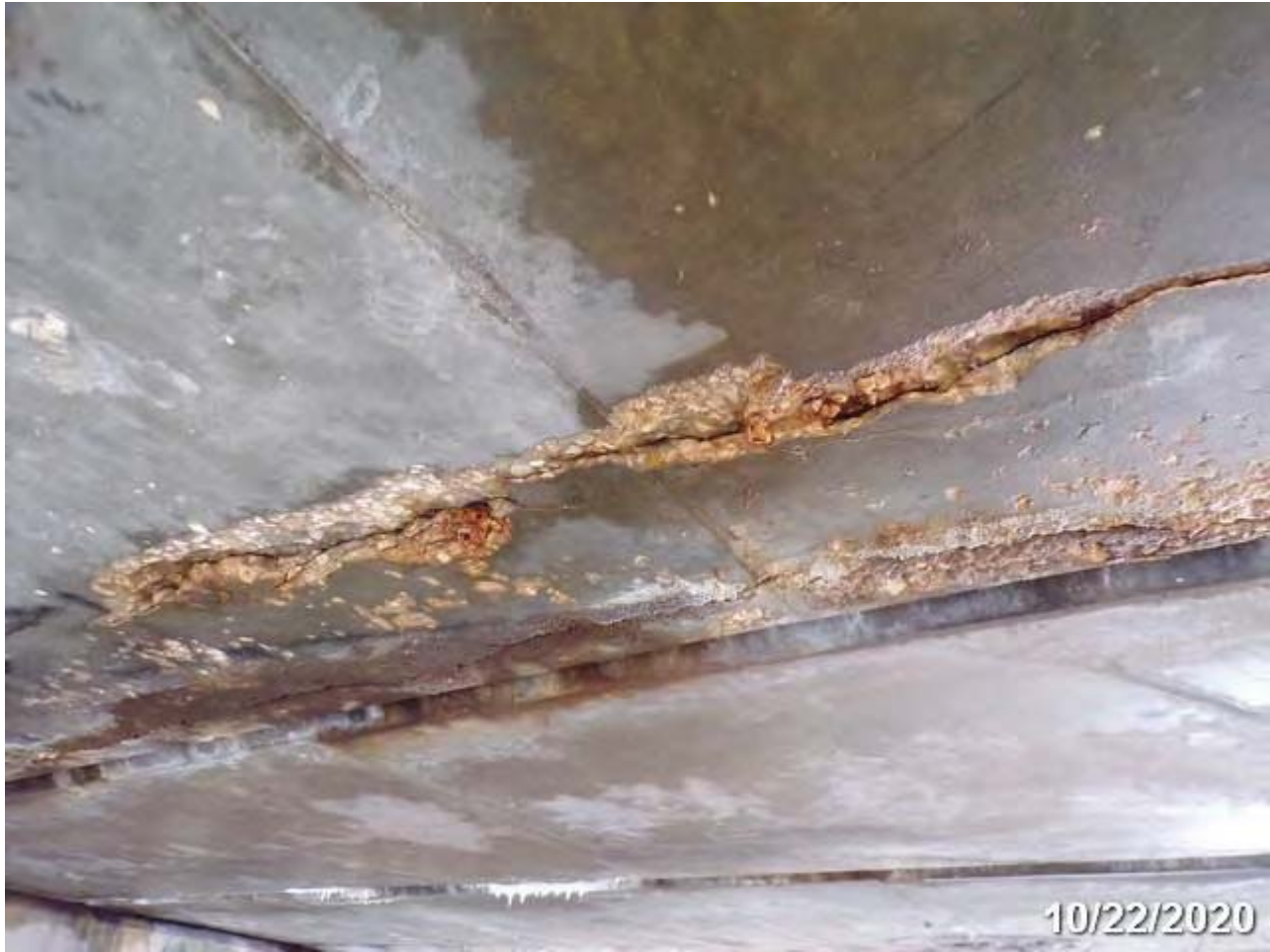
PHOTO 10: ELEMENT/ENV: 8099/3 PS Conc Slab (Sonovoid)
