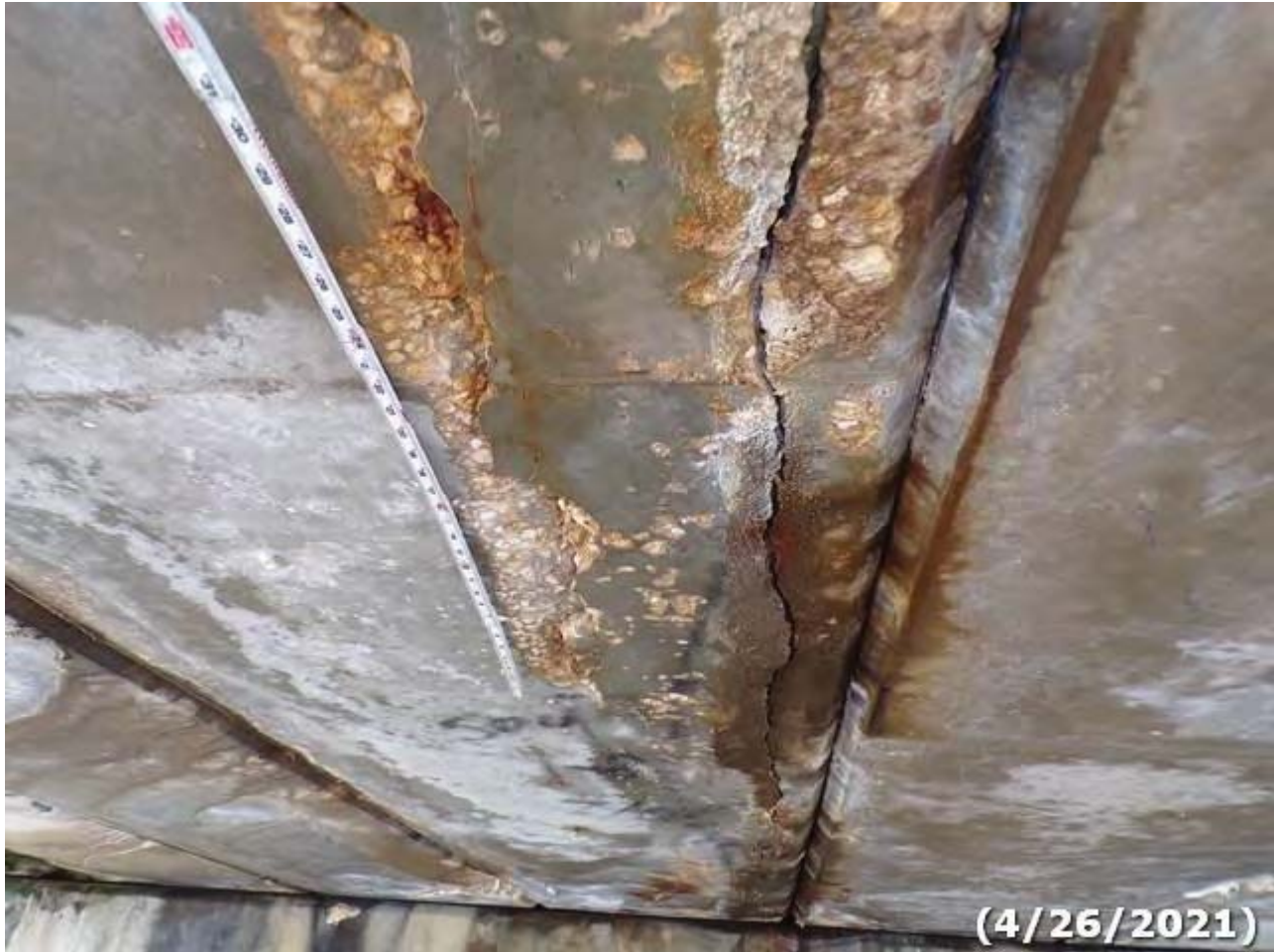
Photo 07 Element/Env 8099/3: PS Conc Slab (Sonovoid)
