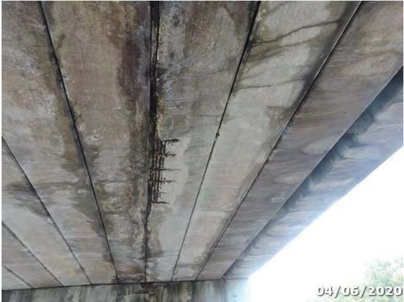
Photo 08 Element/Env 8099/3: PS Conc Slab (Sonovoid)
