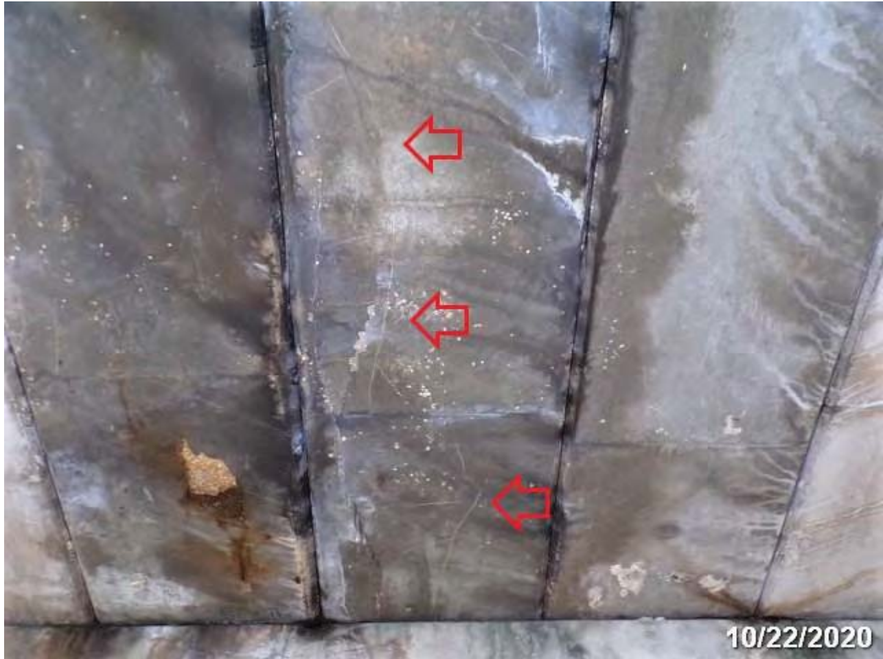
PHOTO 18: ELEMENT/ENV: 8099/3 PS Conc Slab (Sonovoid)
