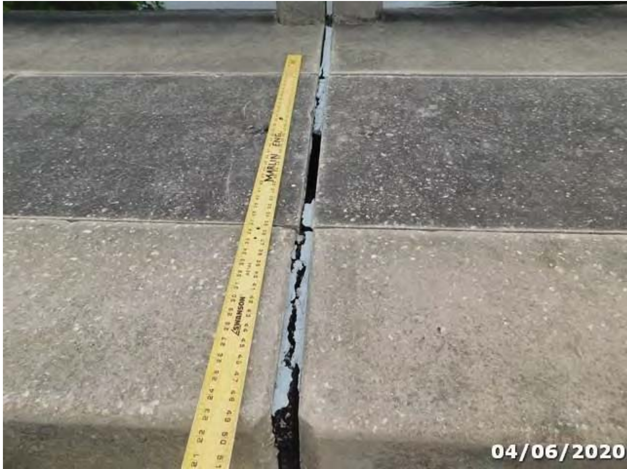
Photo 15 Element/Env 301/3: Pourable Joint Seal
