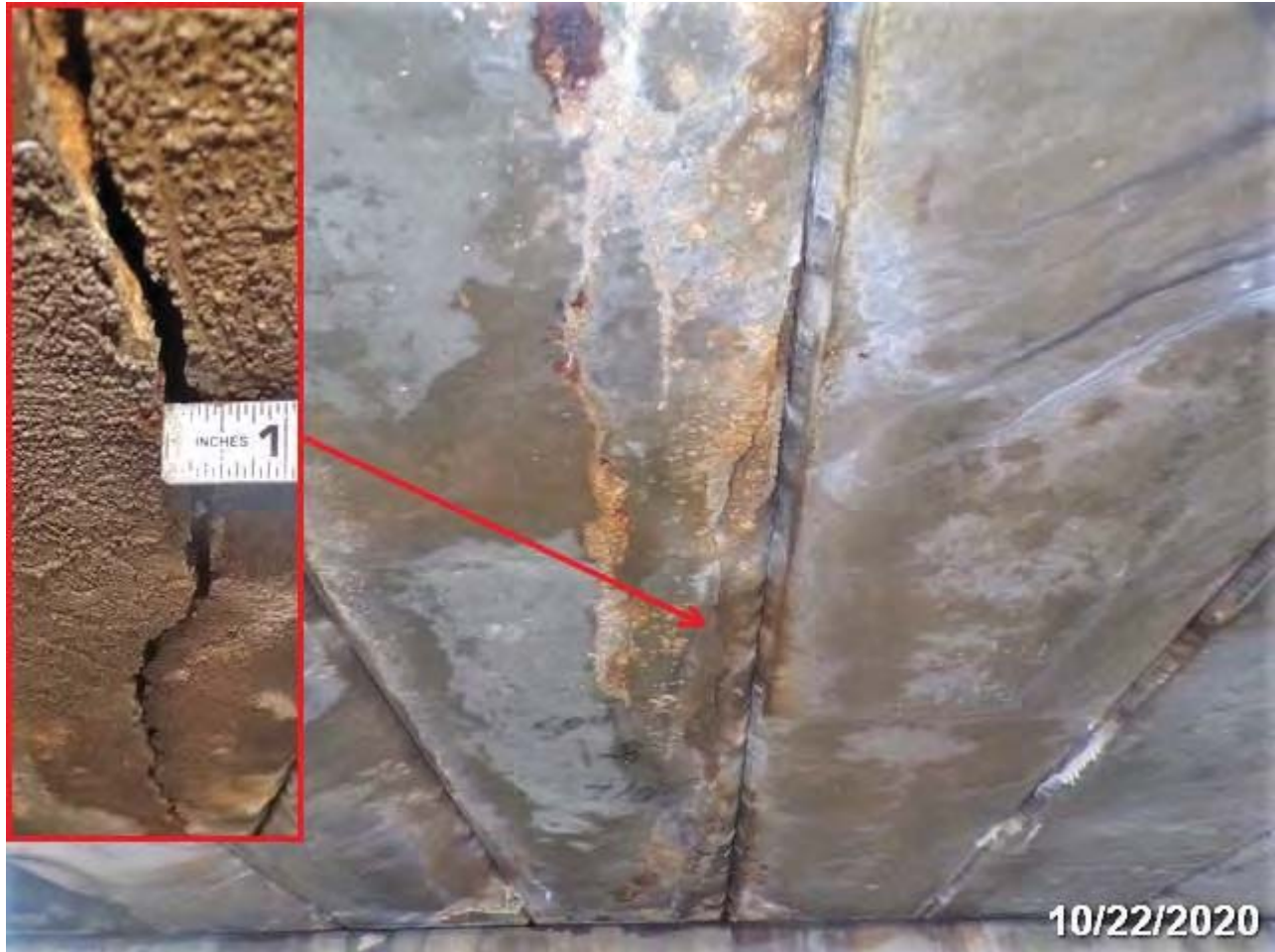
PHOTO 09: ELEMENT/ENV: 8099/3 PS Conc Slab (Sonovoid)
