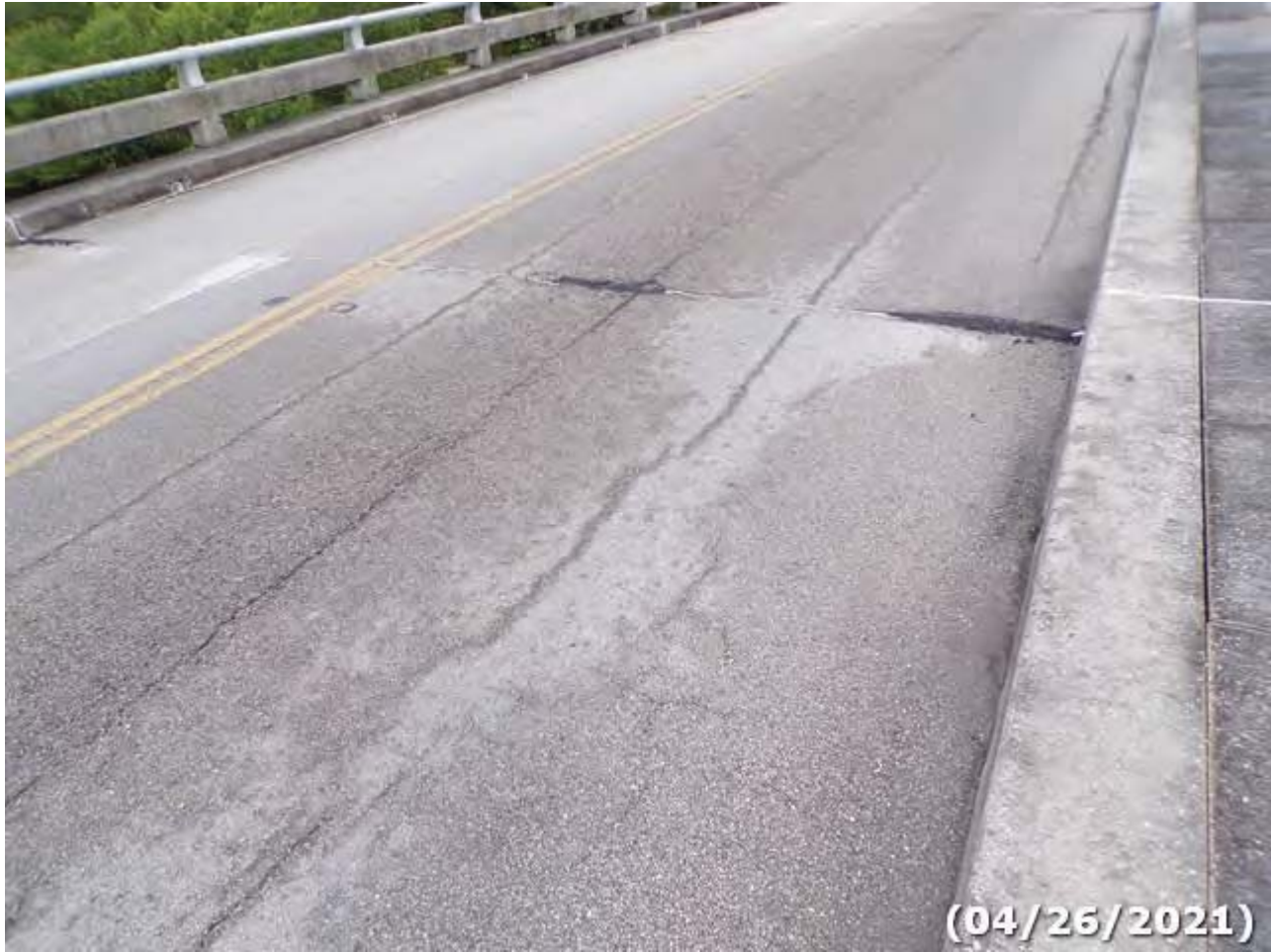
Photo 11 Element/Env 8099/ 510/3: PS Conc Slab (Sonovoid)/ Wearing Surfaces
