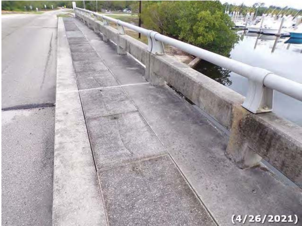
Photo 02 Element/Env 8099/3: PS Conc Slab (Sonovoid)
