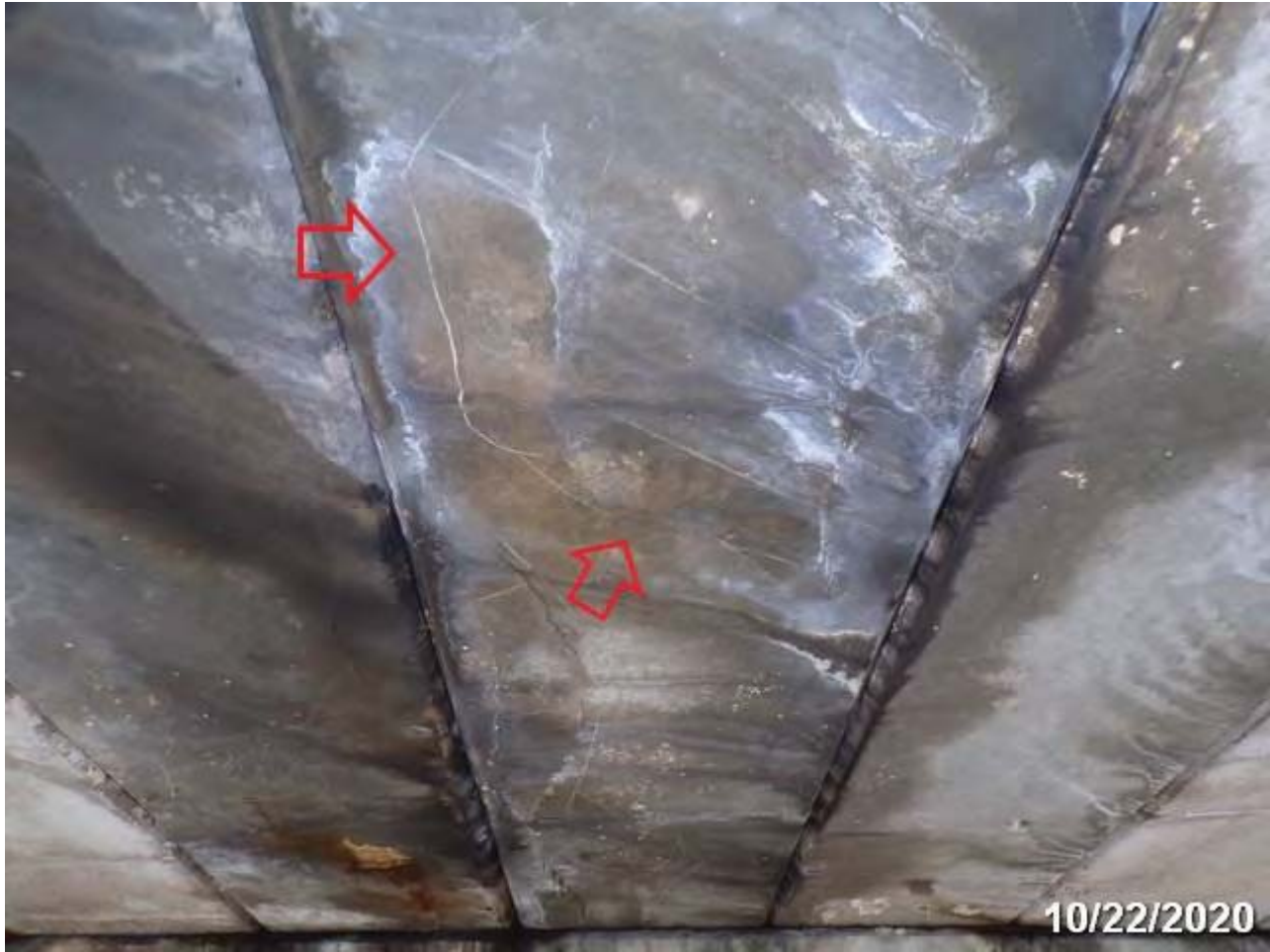
PHOTO 19: ELEMENT/ENV: 8099/3 PS Conc Slab (Sonovoid)
