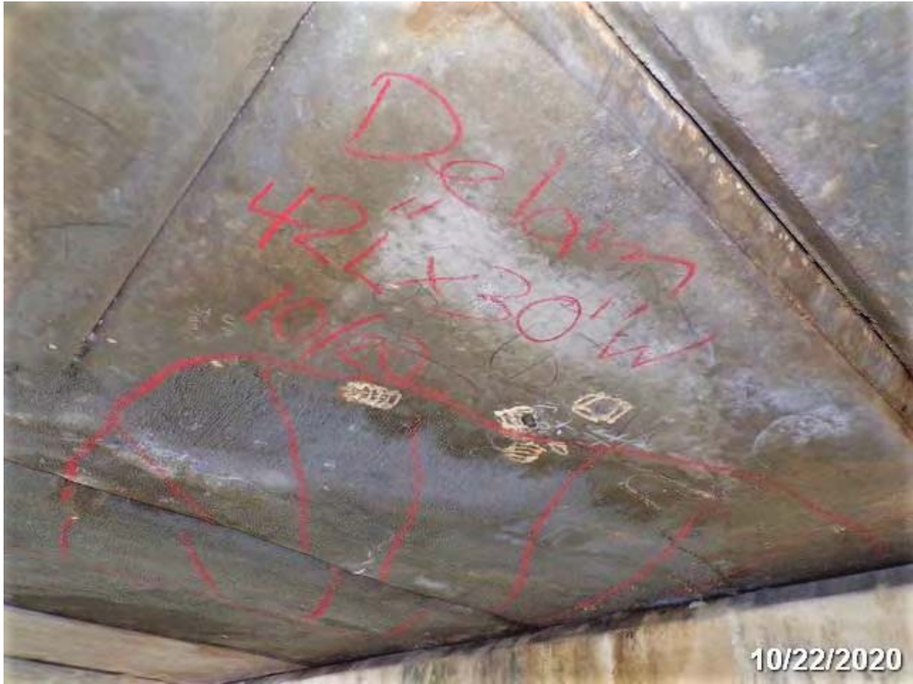
PHOTO 22: ELEMENT/ENV: 8099/3 PS Conc Slab (Sonovoid)
