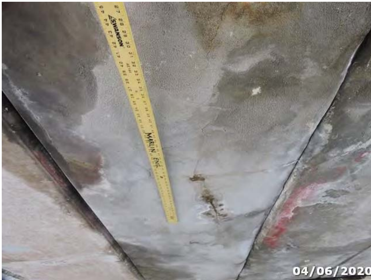
Photo 05 Element/Env 8099/3: PS Conc Slab (Sonovoid)
