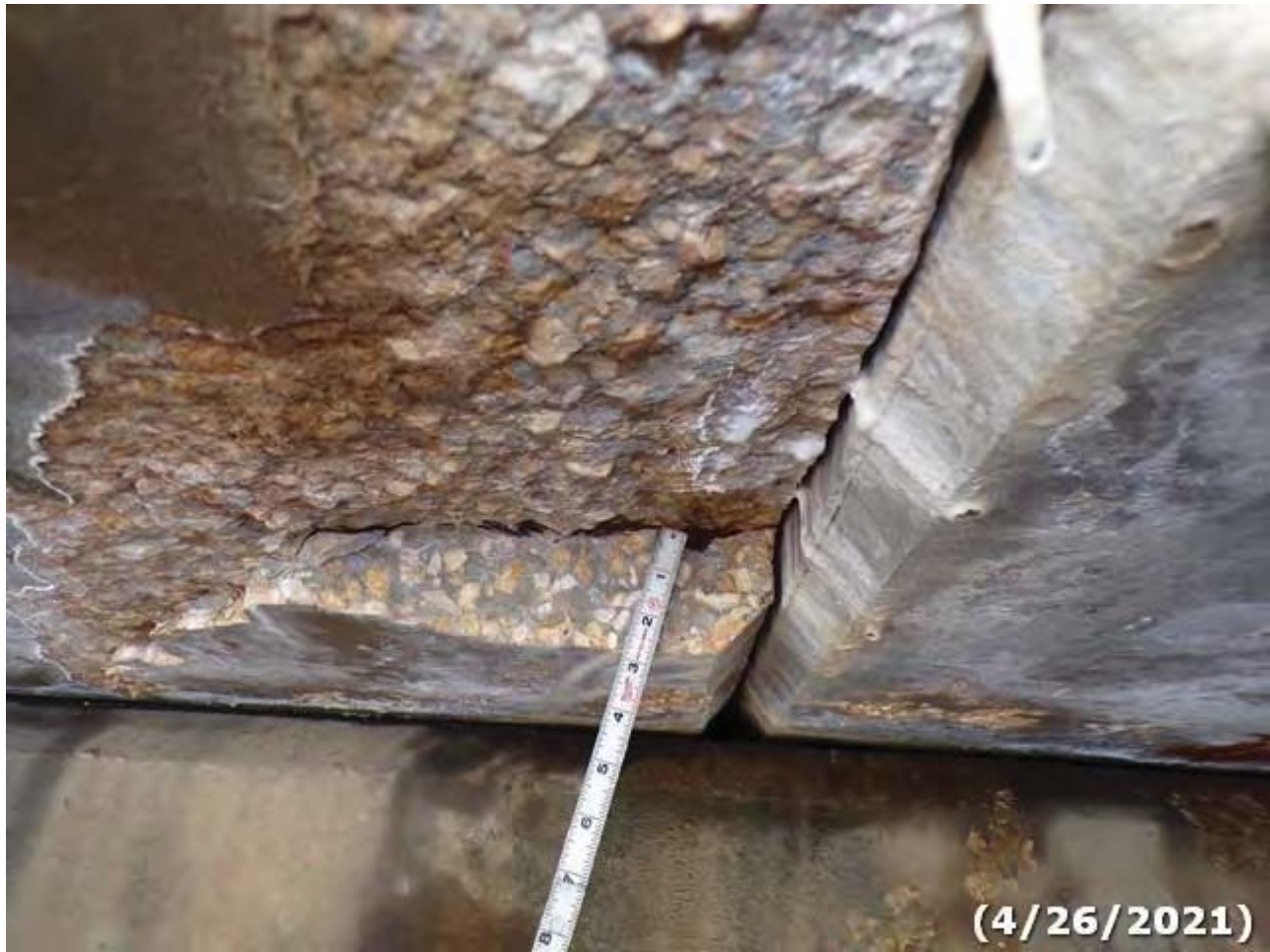
Photo 04 Element/Env 8099/3: PS Conc Slab (Sonovoid)
