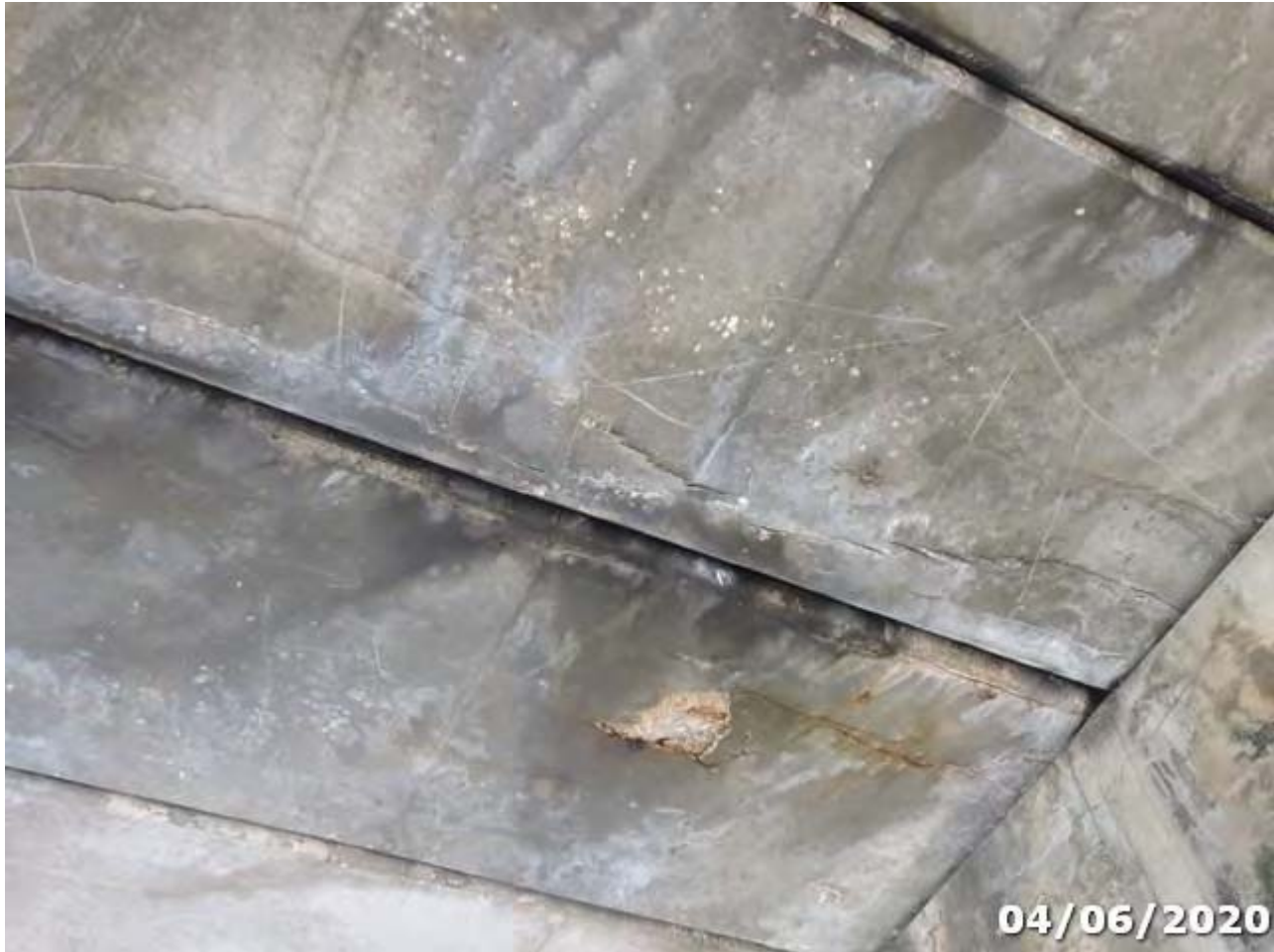
Photo 04 Element/Env 8099/3: PS Conc Slab (Sonovoid)
