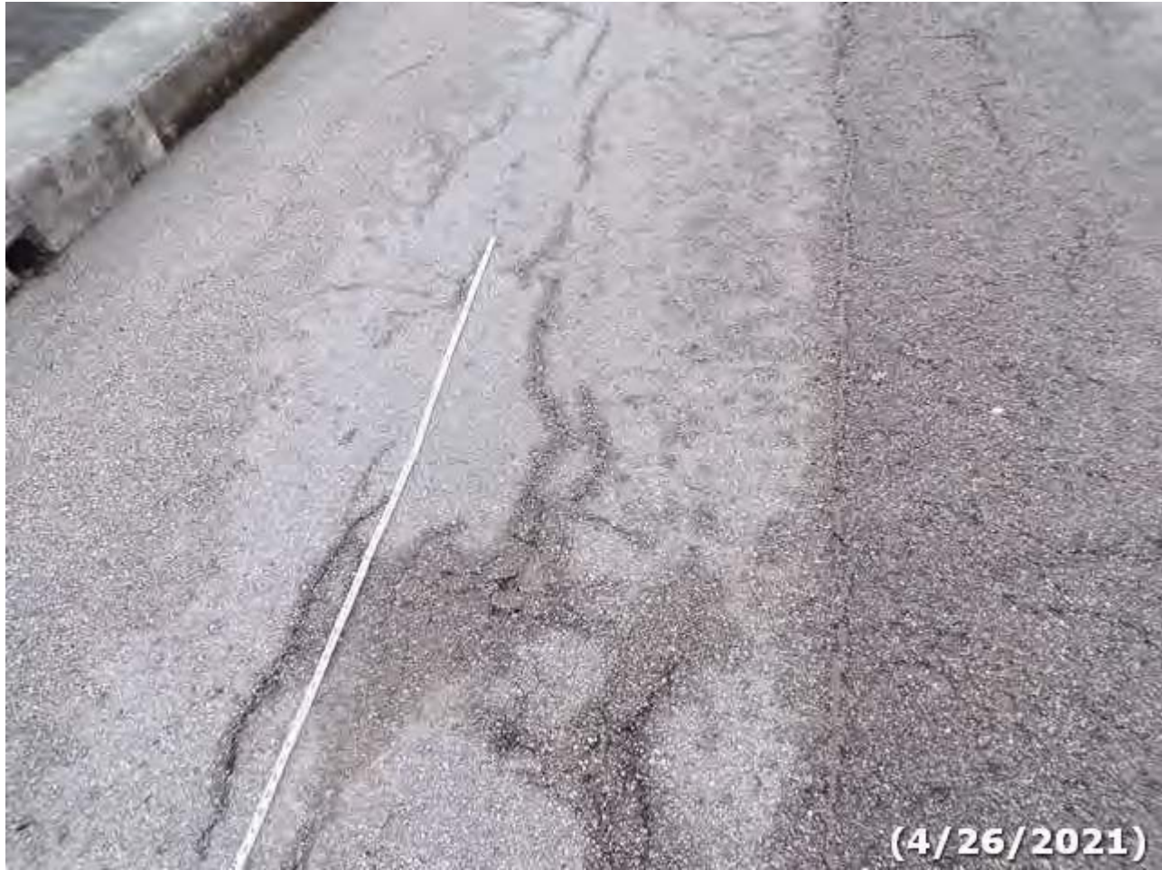
Photo 12 Element/Env 8099/ 510/3: PS Conc Slab (Sonovoid)/ Wearing Surfaces
