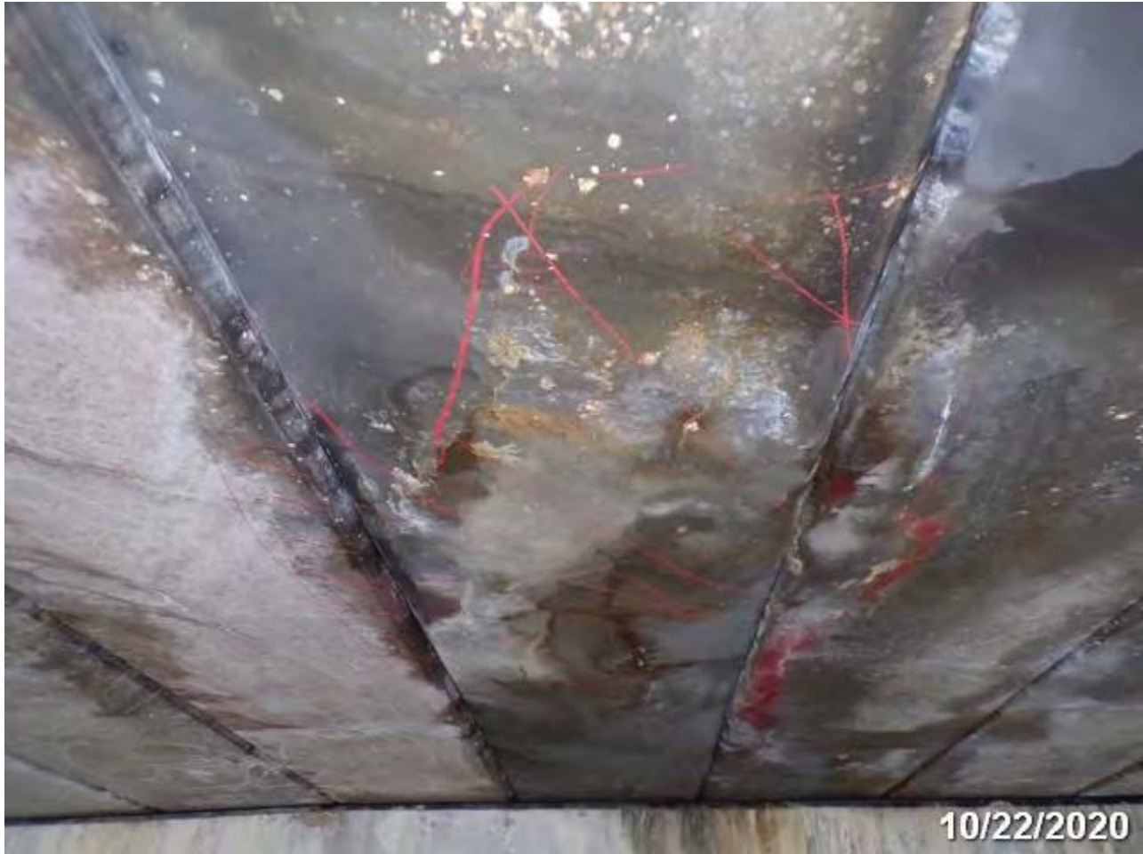
PHOTO 20: ELEMENT/ENV: 8099/3 PS Conc Slab (Sonovoid)
