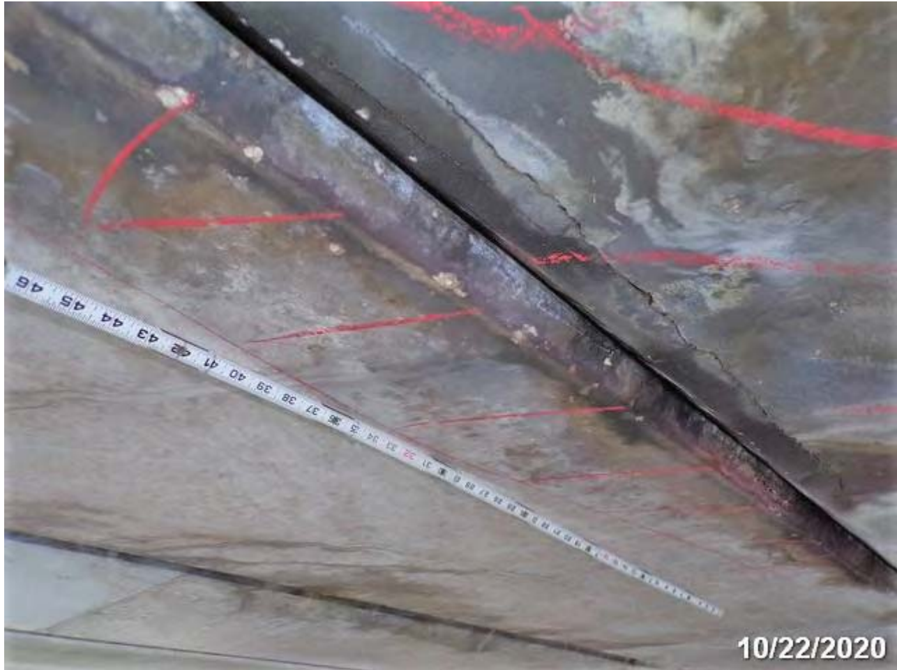
PHOTO 17: ELEMENT/ENV: 8099/3 PS Conc Slab (Sonovoid)
