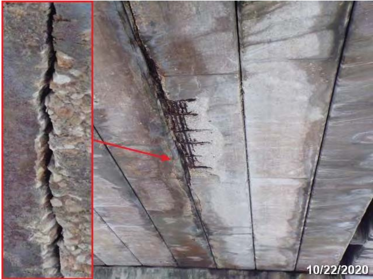
PHOTO 14: ELEMENT/ENV: 8099/3 PS Conc Slab (Sonovoid)
