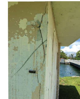
STUCCO DAMAGE EXHIBIT (NE CORNER)
