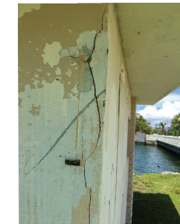
STUCCO DAMAGE EXHIBIT (NE CORNER)
