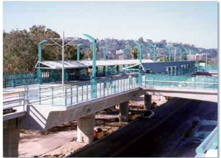
Pre-treatment with compaction grouting for long-term liquefaction mitigation protected the integrity of caissons supporting light rail piers.
