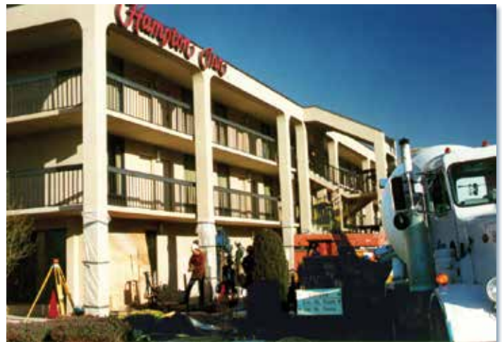
Remedial compaction grouting successfully treated collapsible soils beneath the hotel, reducing future settlement potential to an acceptable level.
