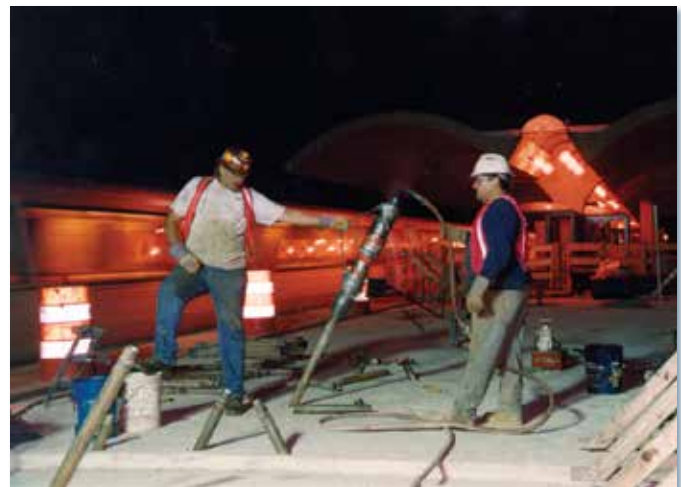
The Denver System of compaction grouting was used to consolidate fill beneath two, settling subway platforms.
