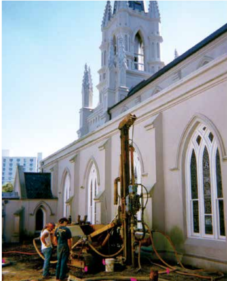
Compaction grouting was used to seal this 160-foot diameter sinkhole that extended down to the Floridan aquifer.
