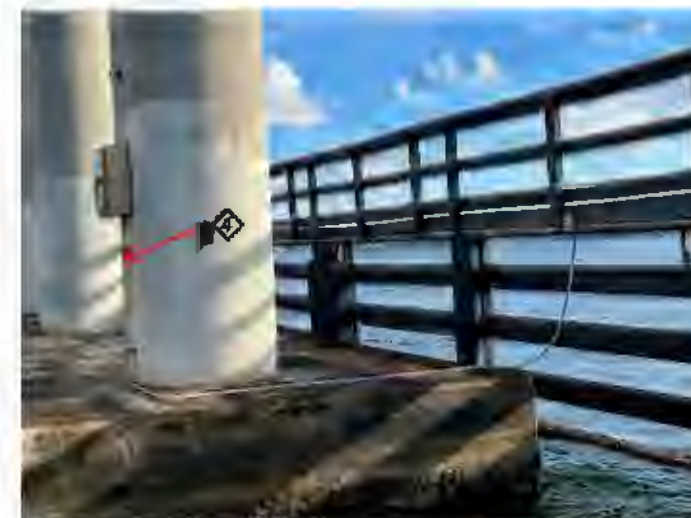
PHOTO 3 - EXISTING WEST FENDER CONNECTION. PROVIDE SIMILAR CONNECTION FROM EAST PIER J-BOX TO EXISTING EAST FENDER LIGHTS.
