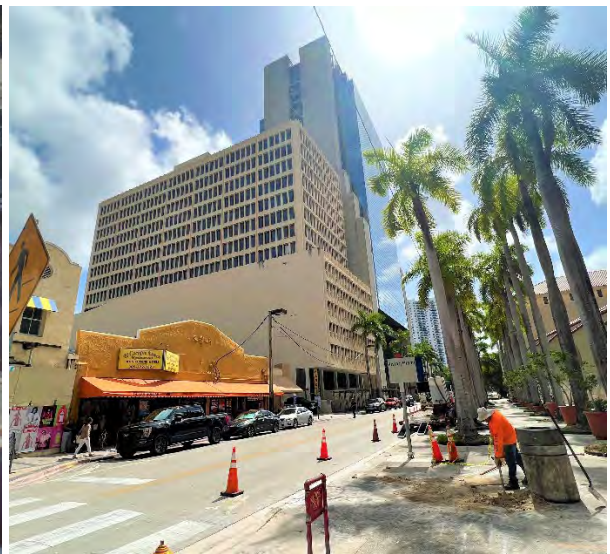
Looking in the southwest toward the north entrance to the 140 W Flagler building
