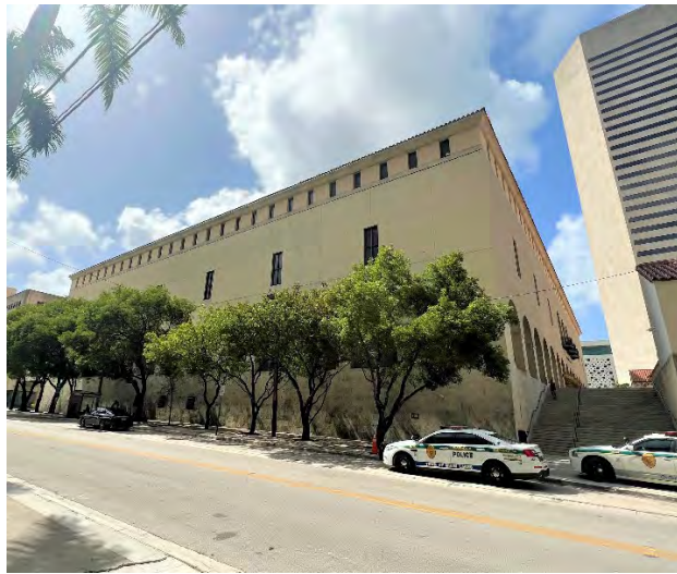
Looking north from W Flagler Street toward the midblock stairs of the Cultural Center
