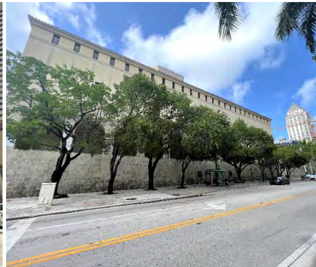
Looking northeast from W Flagler Street toward the Cultural Center Block
