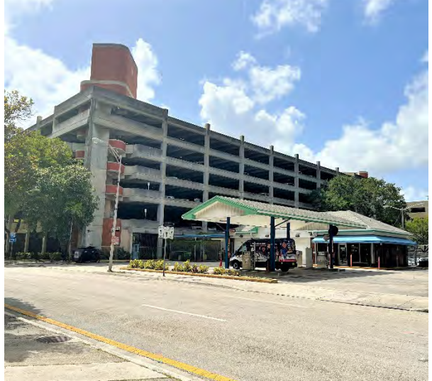
Looking northwest toward the south entrance to the Motor Pool Gas Station
