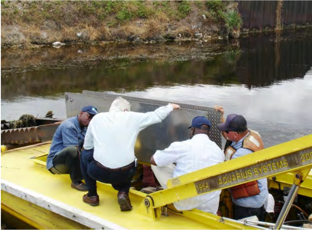
Checking out the diesel engine
