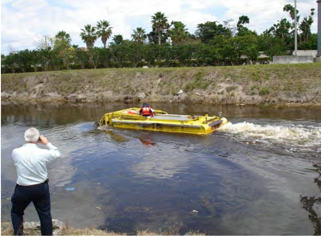
The plow is dragged along the bottom of the canal
