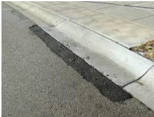
Illustration 2 – Curb and Gutter Work
