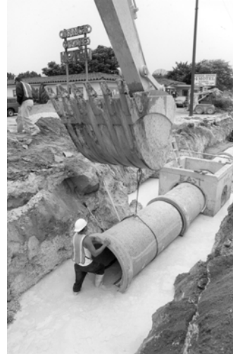
Crews working on installing stormwater drains
