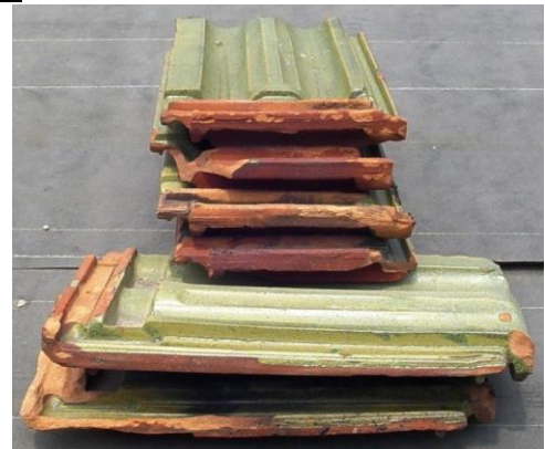
Front View - Staged Tiles (Slope ↓)
